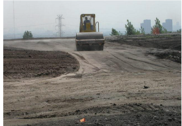
Compaction of PDM grading layer
