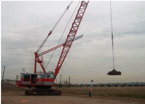
Dynamic compaction of waste
