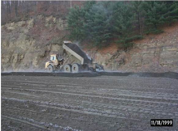
Placing cured PDM in lifts
