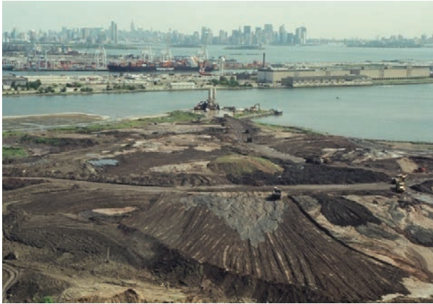
Brownfield remediation with PDM
