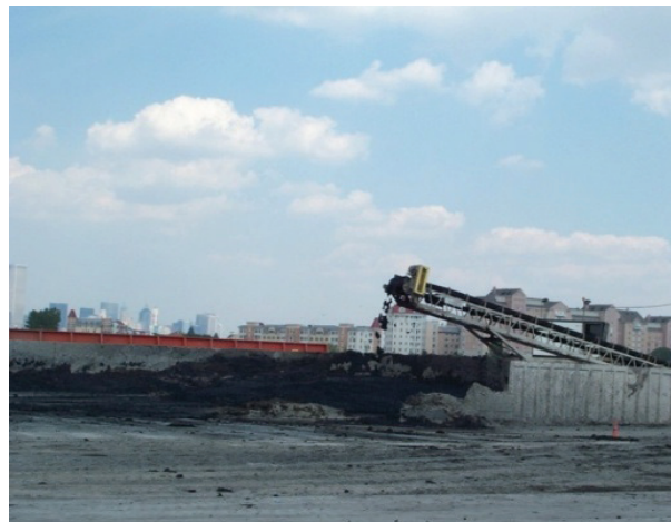
Radial stacker and PDM containment area
