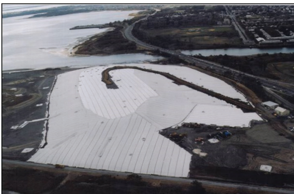
Geotextile membrane on landfill
