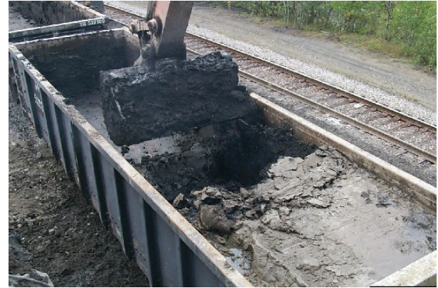
Unloading PDM from rail car
