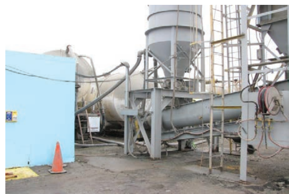
Pneumatic pozzolan metering system
