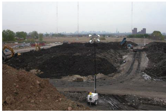
Interim PDM storage facility
