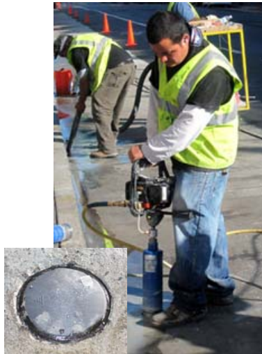
Figure 1: Sensor and sensor installation process –Courtesy of SFpark 2
