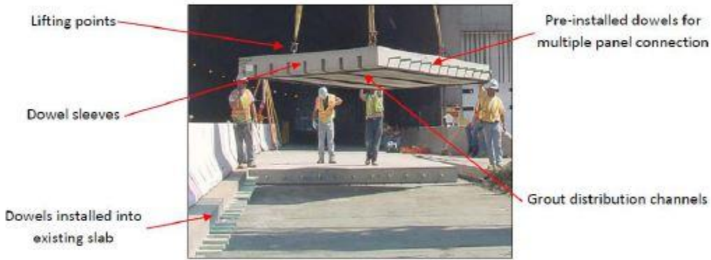
Figure – 4 Installation of Precast Concrete Panel [4]
