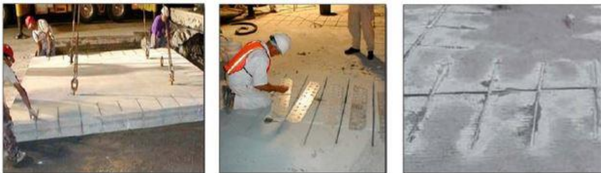
Figure – 8 Fiberglass Tie Installation [6]
