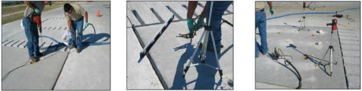
Figure – 9 URETEK Method Installation Technique [3]
