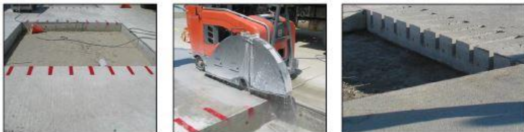
Figure – 13 Dowel Slots Sawing Process [3]
