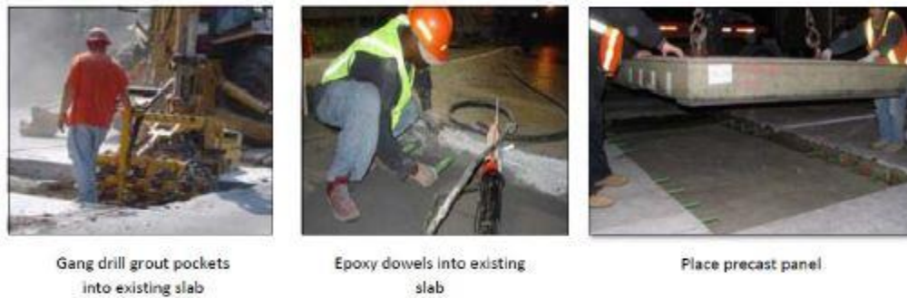
Figure – 2 Preparation of Existing Slab and Installation of Precast Repair Panel [4]
