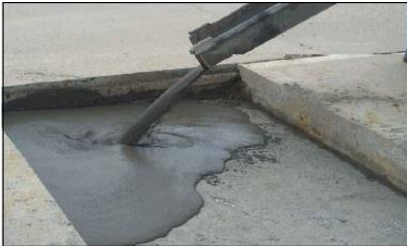
Figure – 6 Flowable Fill Being Place [5]
