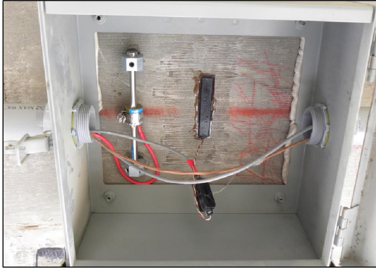
Figure 27: Vibrating Wire & Hitec Strain Gauges
