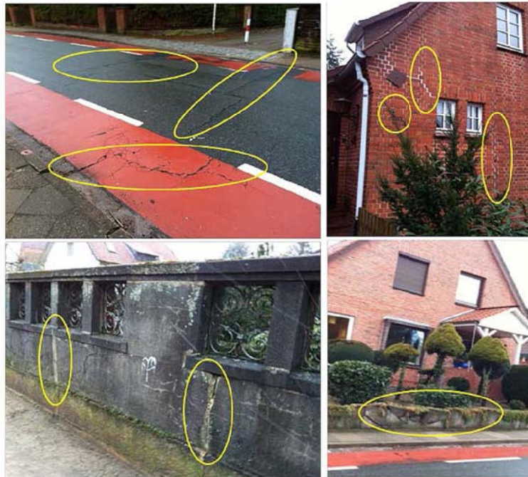
Figure 17. Detection of deformations using Distributed Scatterer Interferometry
