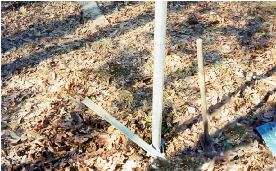
Figure 10 Photograph of driven 2.5 inch line post with one of the anchor blades driven via a sledgehammer into position.
