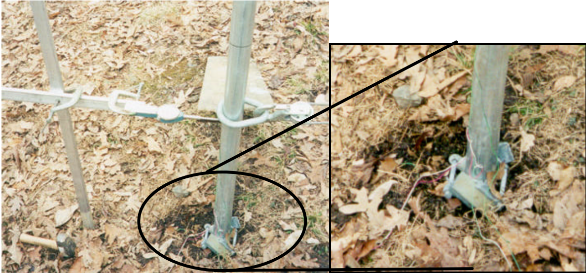
Figure 11 Photograph of fully installed 2.5 inch line post and anchor blades ready to be tested.
