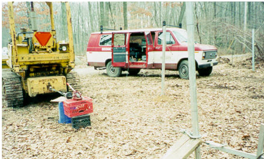
Figure 15 The pull-out system is shown just after beginning a pull-out test.
