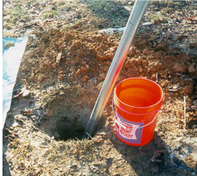
Figure 7 First hole dug on-site for a 2.5 inch line post set in a concrete footing.
