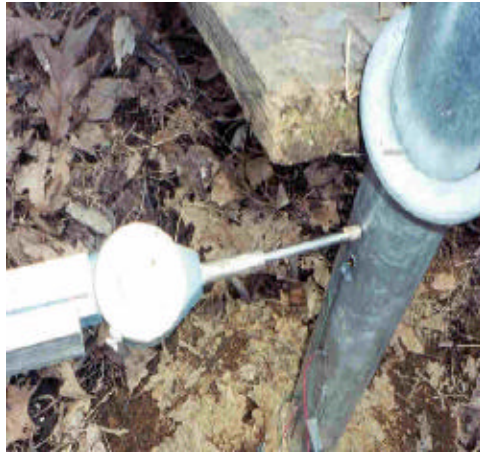
Figure 14 The deflectometer was attached to a stationary pole that was driven in the ground nearby so the deflection could be measured at the pull height.
