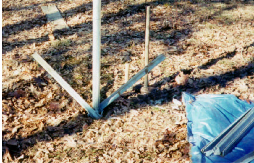
Figure 9 Photograph of driven 2.5 inch line post with one set of anchor blades positioned for installation.
