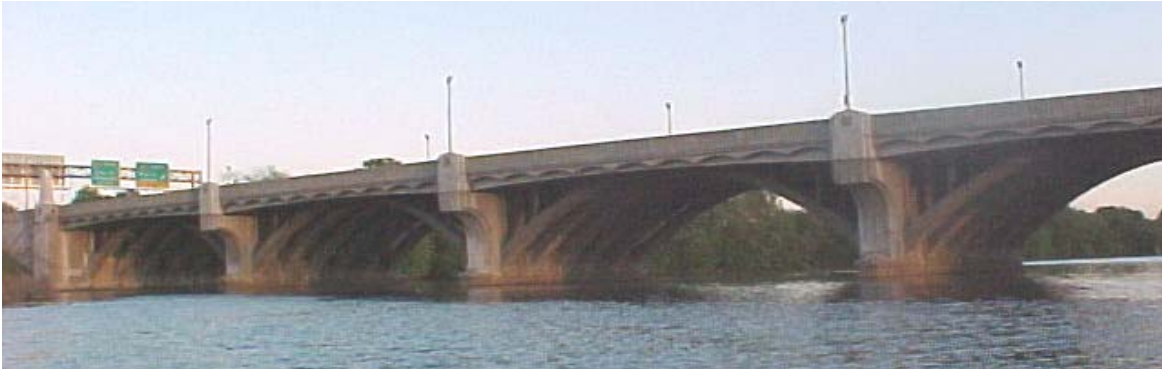
Figure 22. Route 46 Passaic Bridge at Elmwood Park, North Elevation.
