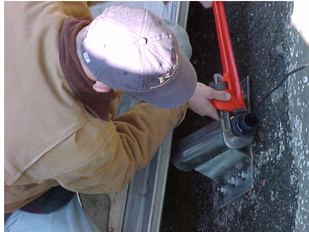
Figure 11. Placing sonar in stainless steel conduit
