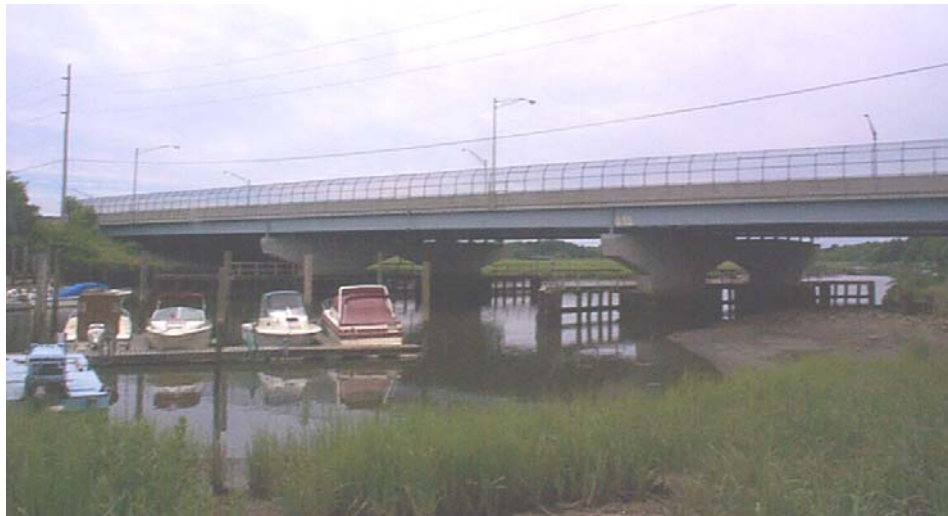
Figure 5. Matawan Bridge North Elevation.
