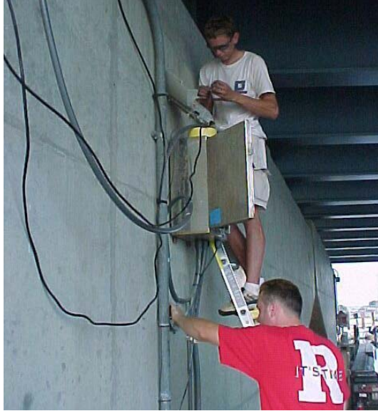
Figure 53. Matawan Bridge Repairs. Aug 2001.
