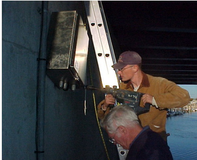
Figure 15. Installation of datalogger by Rutgers and ETI staff.
