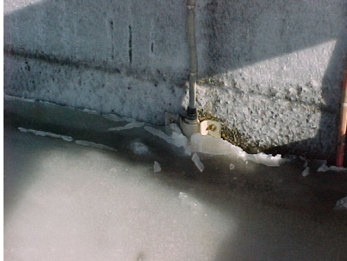
Figure 18. Sonar surrounded by ice. Matawan Bridge, Feb 2000.
