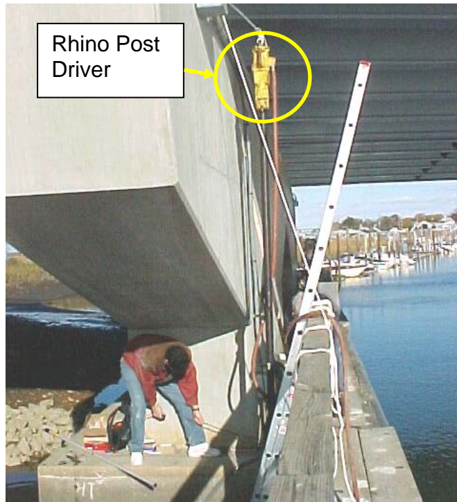
Figure 13. The Rhino™ Post Driver on top of the steel pipe to drive the stainless steel MSC pipe into riverbed.
