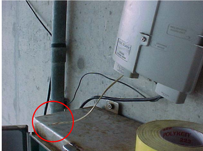
Figure 51. Matawan Bridge Vandalism. Aug 2001. Severed telephone cable and dismantled telephone box
