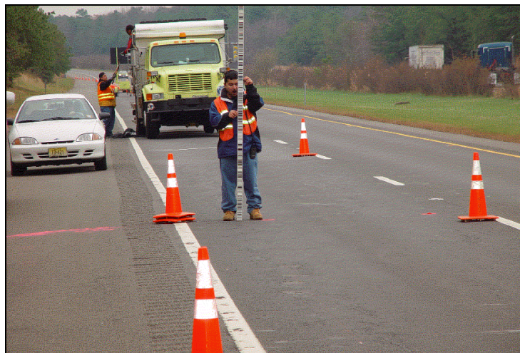
Figure 7. Rod and Level Survey.
