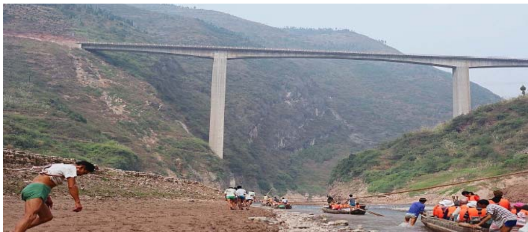
Figure 13: Vulnerability of bridge piers in remote areas.
