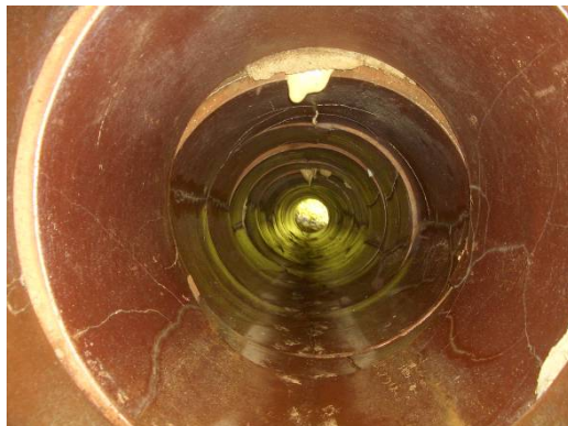
Figure 4. Clay pipe culvert: view of interior
