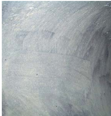
Figure 5. Clay surface coated with inorganic polymer composite
