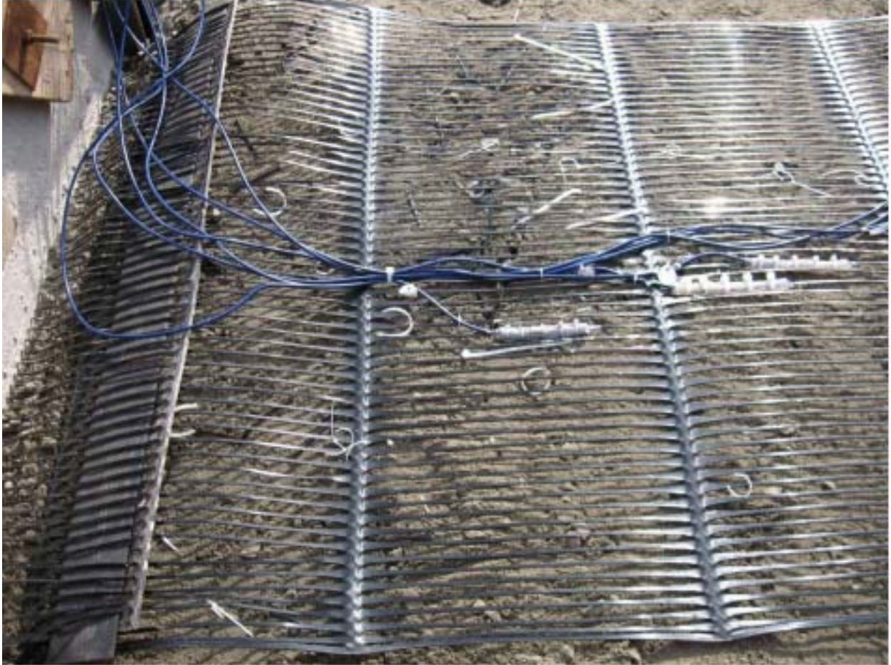
Figure 21. Instrumented Geogrid with Strain Gages
