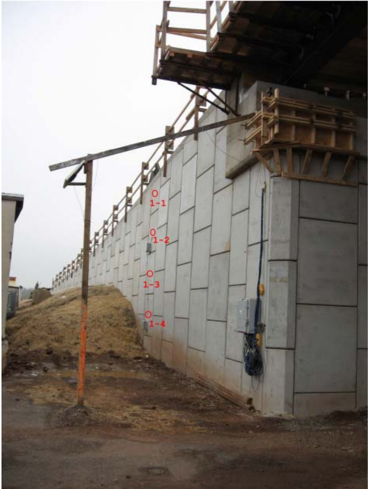
Figure 14. Optical Prism Locations at Wall 1
