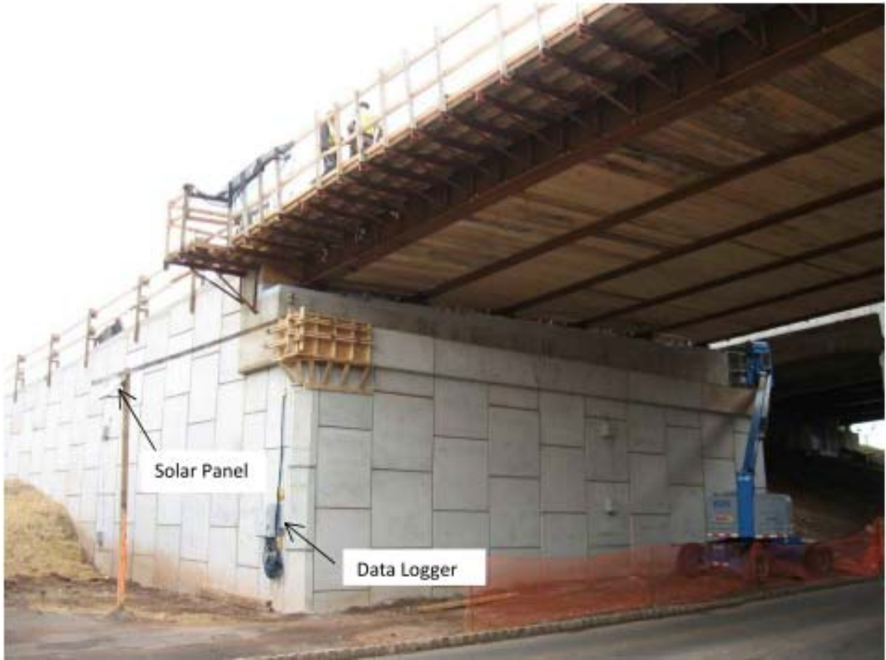
Figure 23. Wall 1 and Wall 3 at End of Construction
