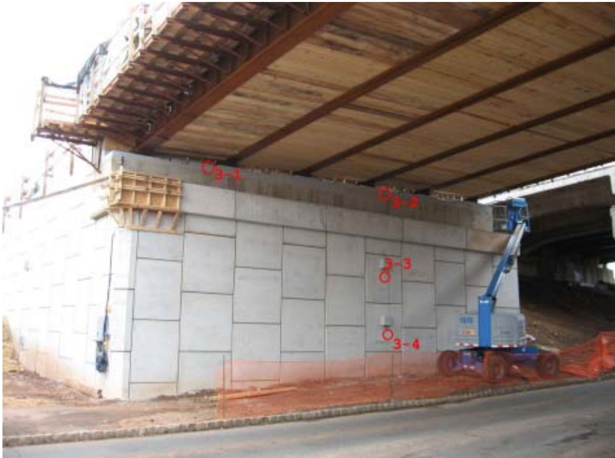
Figure 15. Optical Prism Locations at Wall 3
