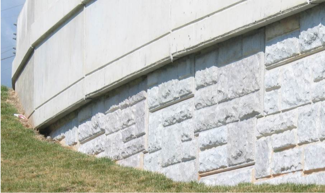
Figure 7. Condition after Application
