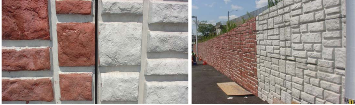
Figure 2. Contrast between Parent and Coated Surfaces
