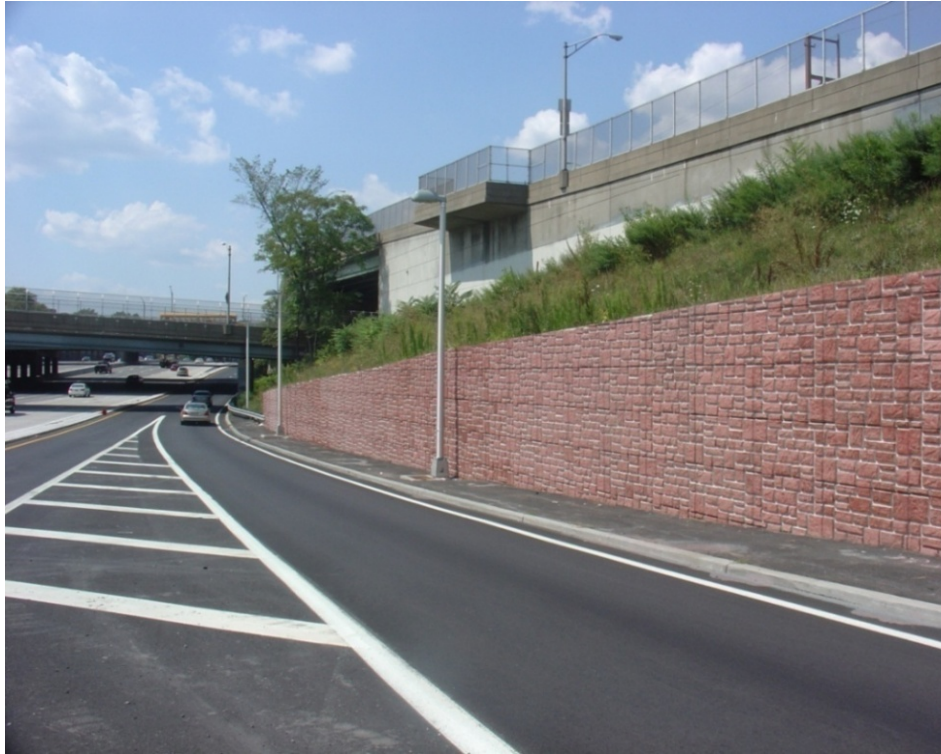
Figure 4. Condition After Coating
