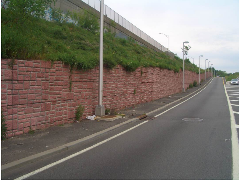
Figure 5. Condition after 1 - 2 Years
