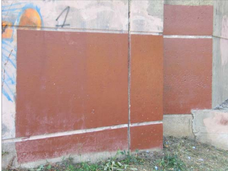
Figure 10. Coated Milltown Bridge Abutment
