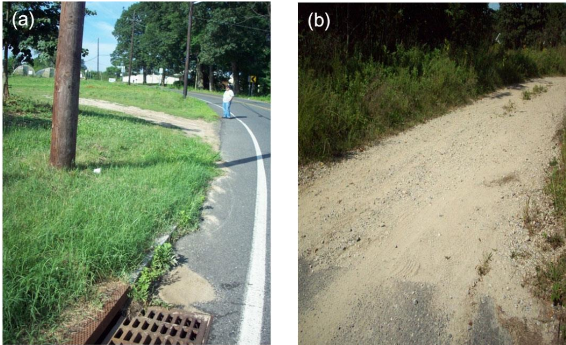
Figure 29. Eroded sand into network: (a) Sand was eroded from the driveway to the farm, (b) Sand was eroded from the driveway to the construction area
