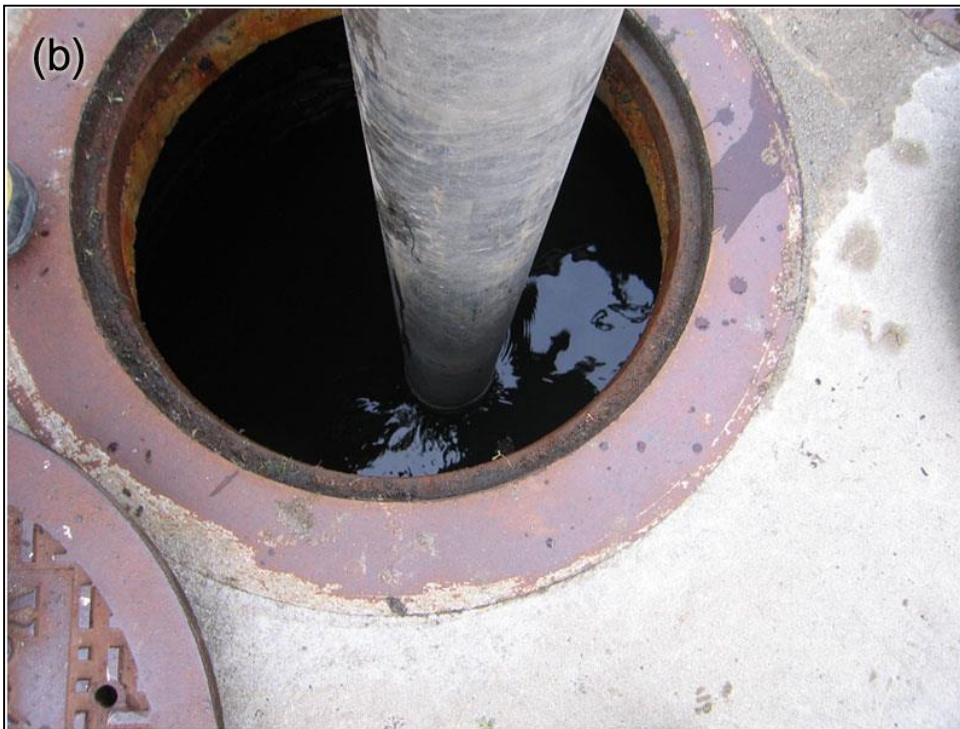
Figure 5. The cleanout of the Vortechs system: (a) Cleaning out the Vortechs unit with vacuum truck, (b) Pumping out water first and then pumping out solids (Typically)
