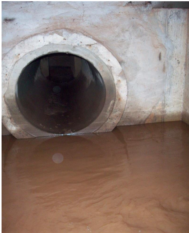
Figure 28. No flow from diversion chamber to treatment device (Point B in DC 1 in Figure 25).
