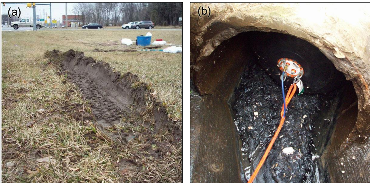
Figure 6. Encountered problems while cleanout at RU14-01 site: (a) Soft ground might not support the vacuum truck after a rainy day. Operation was completed on a dry day, (b) Water was flowing from inlet pipe which size is 42-inch. Operation was completed with a pneumatic pipe plug
