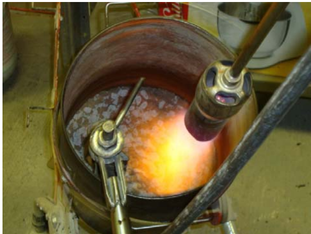
Figure 8 – Heating and Mixing Aggregate Blends
