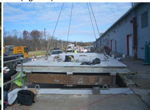
Figure 2: Monitoring during lifting in place
