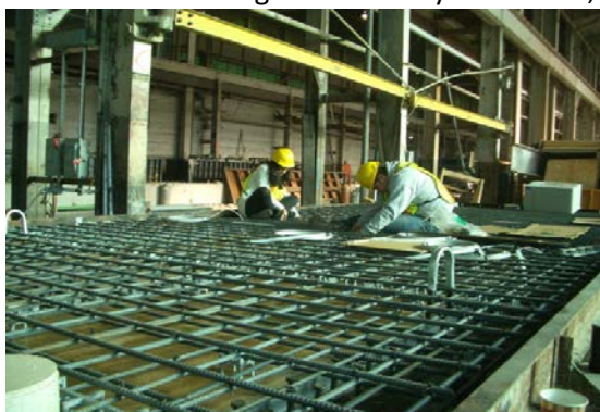
Figure 1: Installing sensors on concrete rebar
