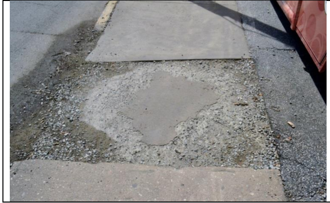
d.) Spalling of sidewalk sections
