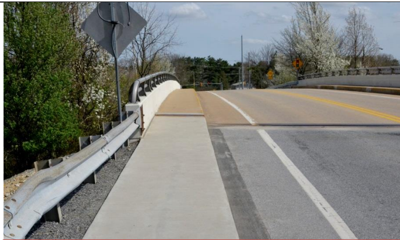
No railing or barrier separating the road from the sidewalk
