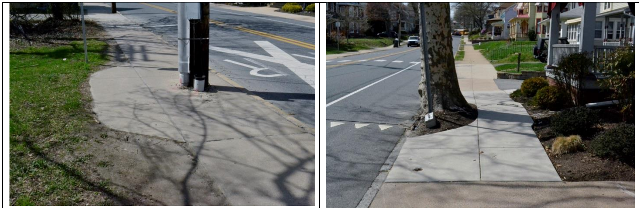
Figure 7: Sidewalk Retrofitting in Newark, Del.
