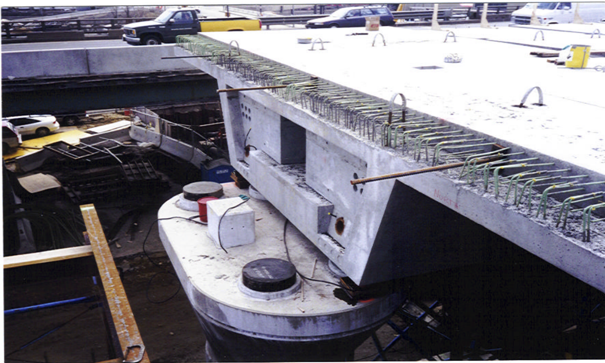
Figure 1. Circular elastomeric bearings used in concrete box girders in Massachusetts.
