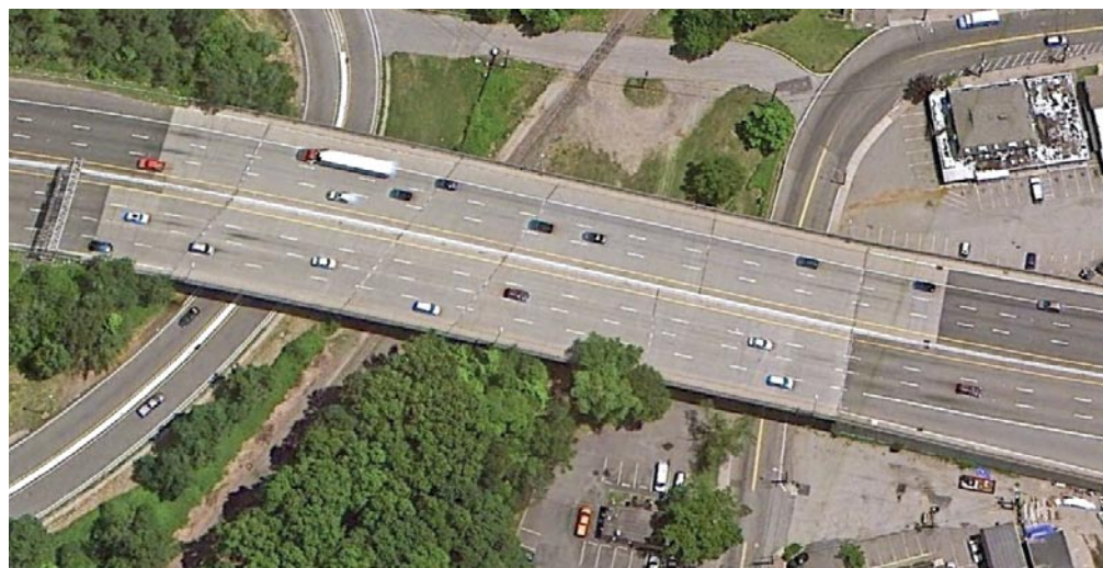
Above: This aerial view of the IBS bridge shows the combination of straight and skewed spans that, among other characteristics, made it ideal for the study.
