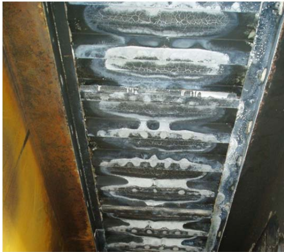
a. Sagging of Stay-in-Place Forms
