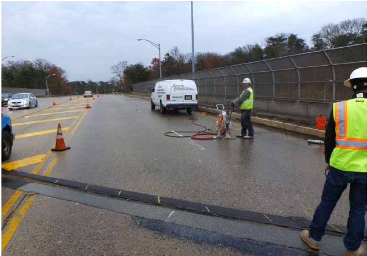
Figure 1. Image of the NDE surveyed area of Creek Road over I-295 Bridge.
