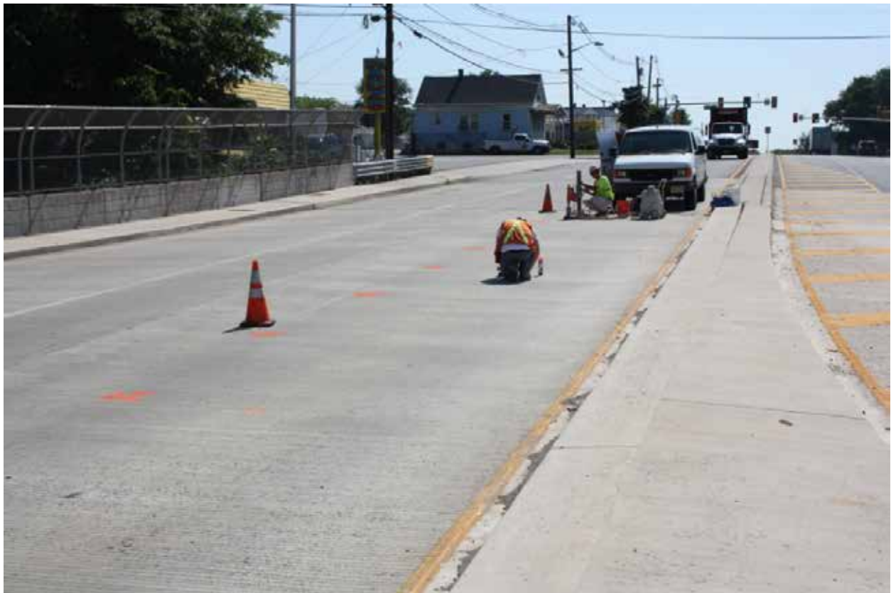
Figure 1. View on the area of Smith Street Bridge surveyed.
