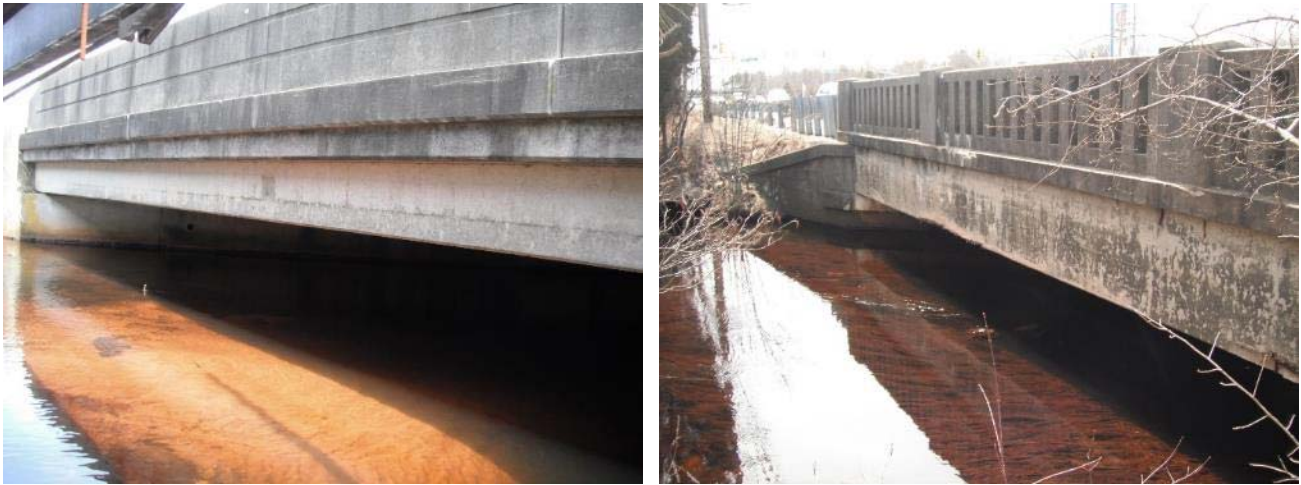
Figure 37: Overview of Structure 1512152 – NJ72 over Mill Creek
