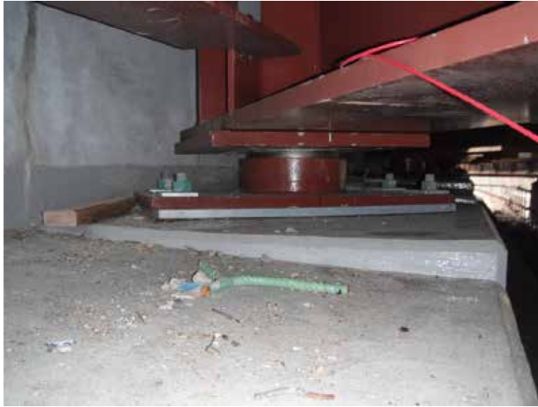
Figure 3: Multi-rotational Pot Bearing
