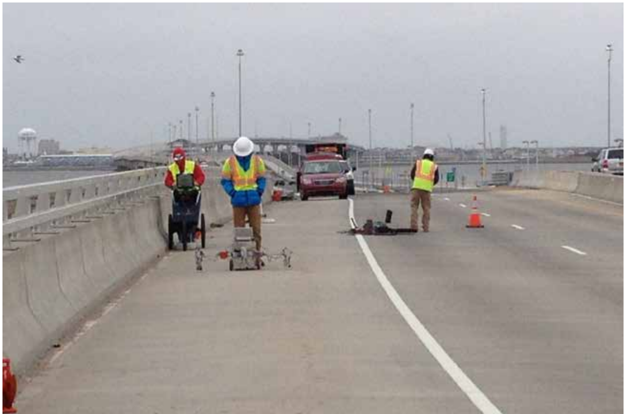
Figure 1. NDE surveys on Route 52 Elbow Creek bridge deck.
