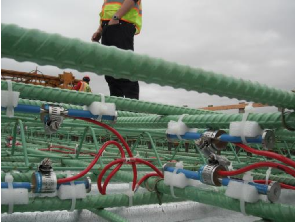
Figure 40: Vibrating Wire Embedment Gage Installation at Route 3 over NJ Transit
