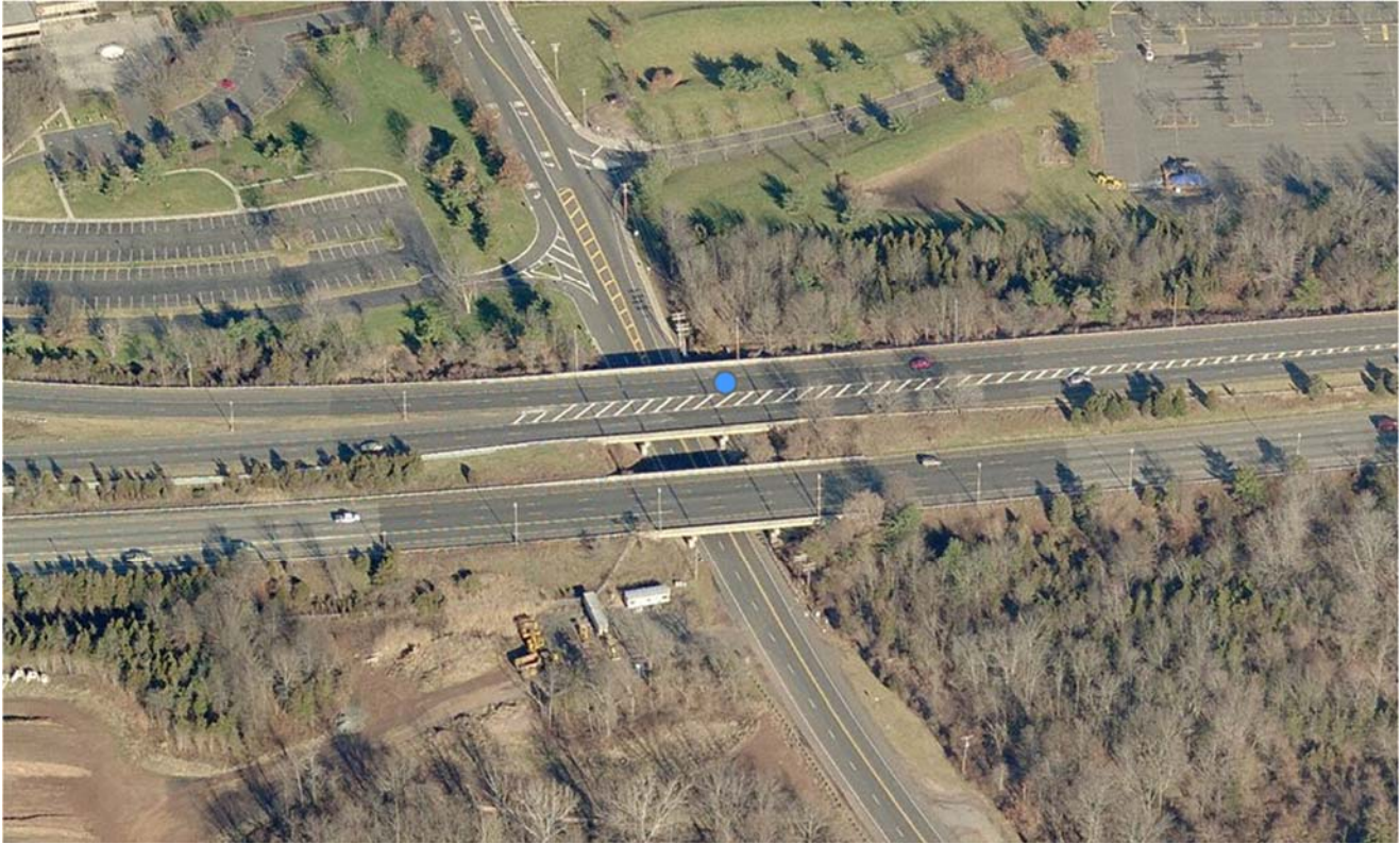
Figure 8: Structure No. 1817156 Aerial View
