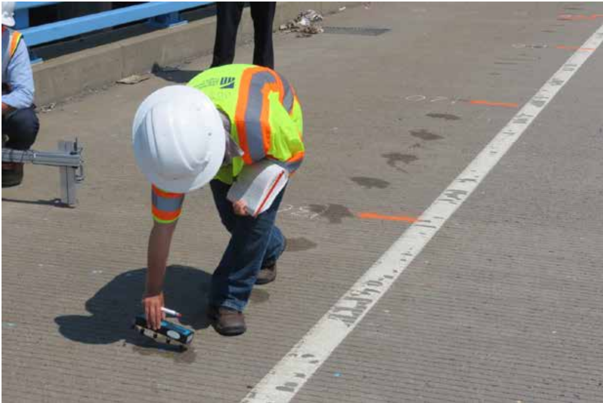
Figure 1. Electrical resistivity measurement on Route 9 Northbound Bridge deck.
