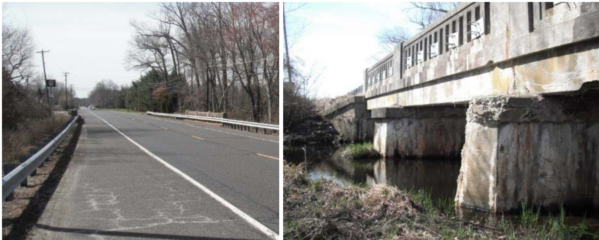
Figure 34: Overview of Structure 0324152 – US206 over Springers Brook
