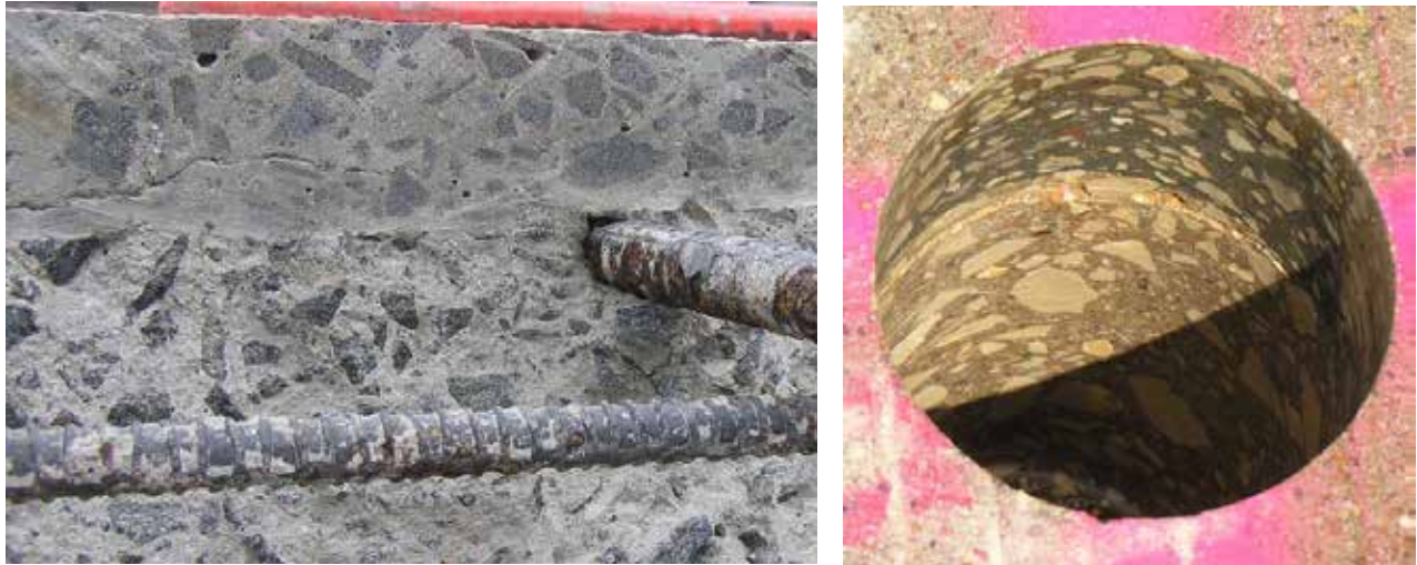
Figure A5. Initial (left) and progressed delamination (right).
