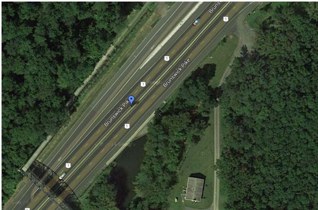
Figure 54: Structure 1103152 – Aerial View
