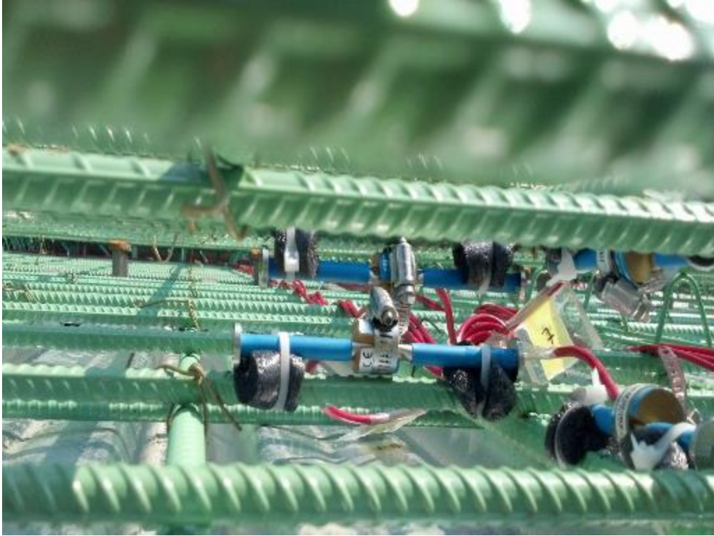
Figure 66: Vibrating Wire Embedment Gage Installation at Collings Ave
