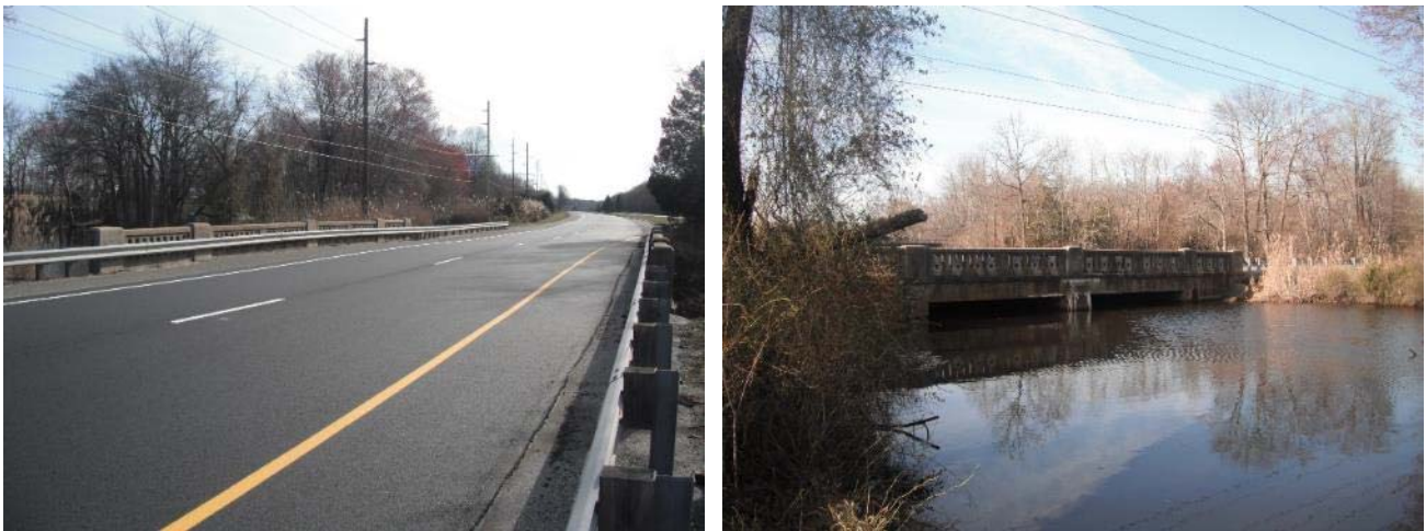
Figure 68: Structure 1701151– US40 over W. Branch of Game Creek
