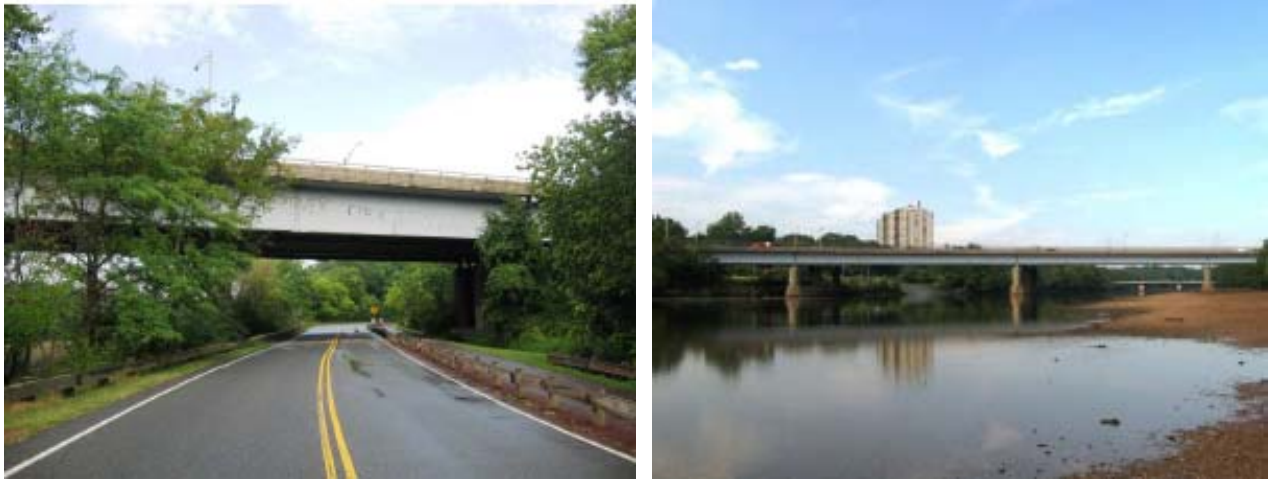
Figure 58: Structure 1237155 – NJ18 over Raritan River
