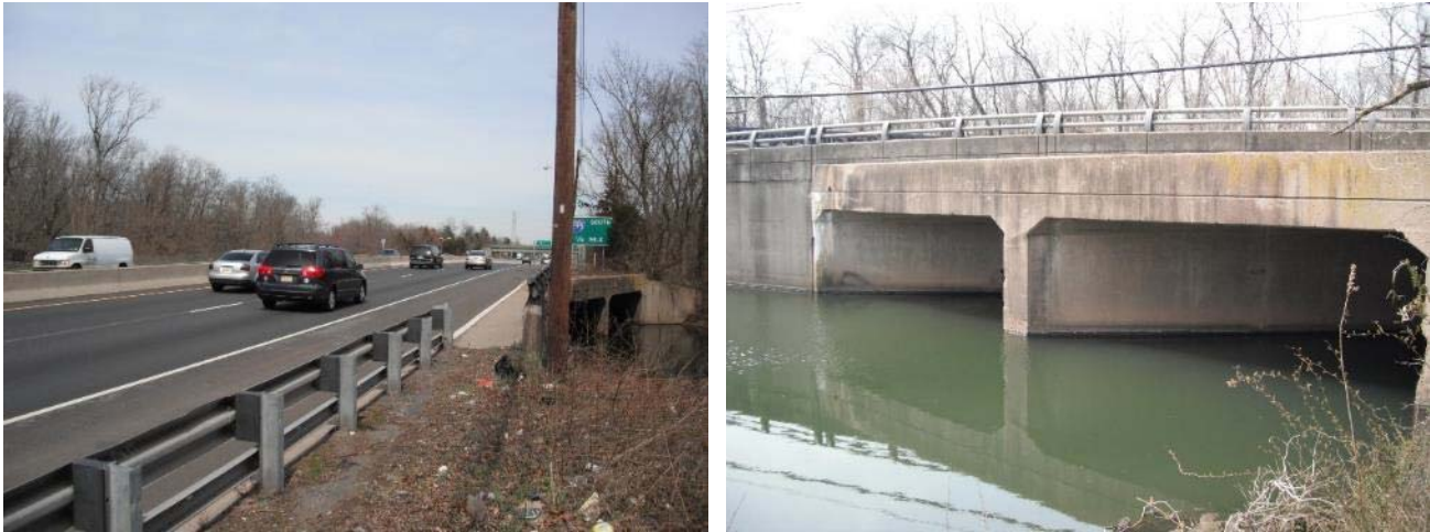
Figure 53: Overview of Structure 1103152 – US1 over D&R Canal
