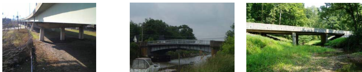
Figure 3. Photos of (a) viaduct bridge, (b) former bascule bridge, and (c) prestressed spread box girder bridge
