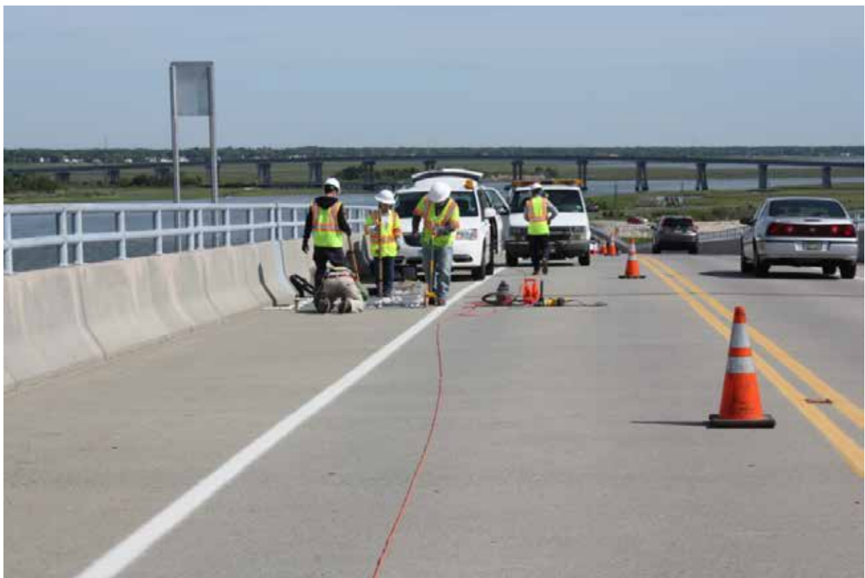
Figure 1. Preparation for NDE surveys on Ocean City Longport Bridge.
