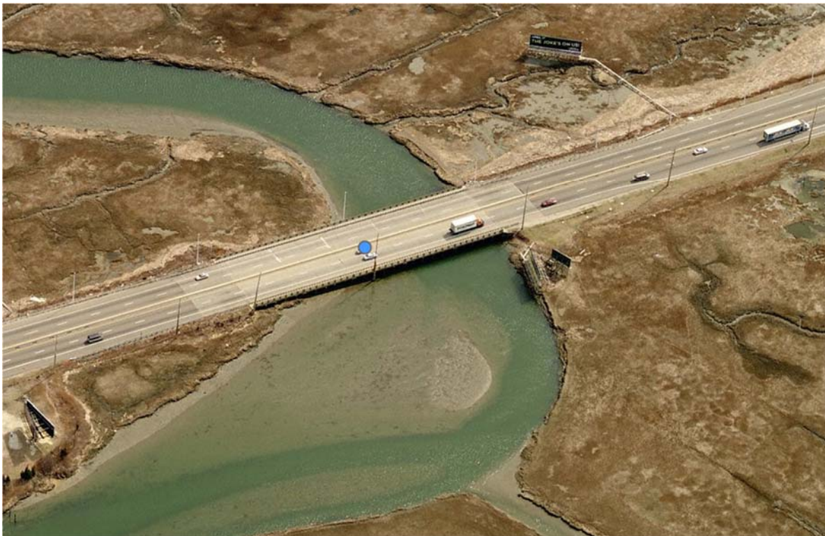
Figure 14: Structure No. 0103150 Aerial View
