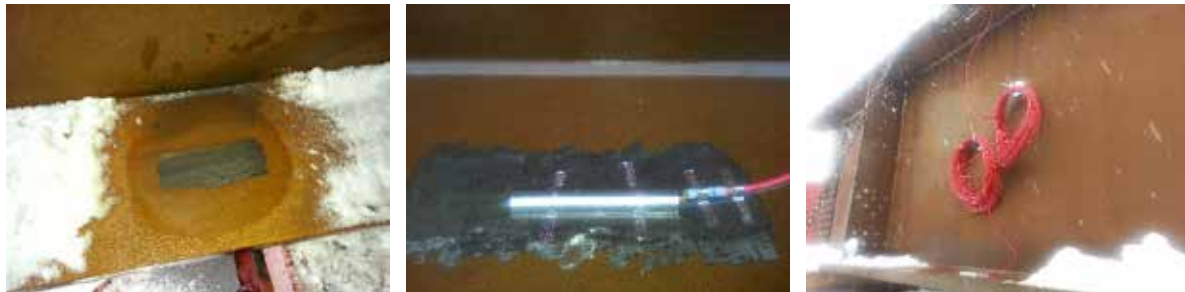
Figure 15: Strain Gage Installation
