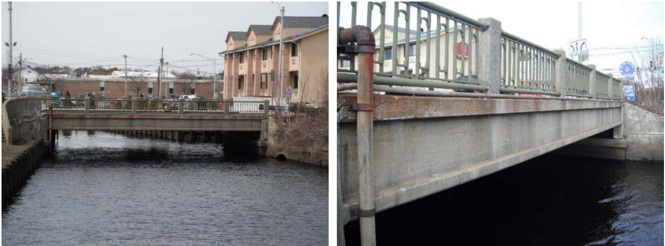
Figure 44: Overview of Structure 1516152 – NJ166 over Toms River
