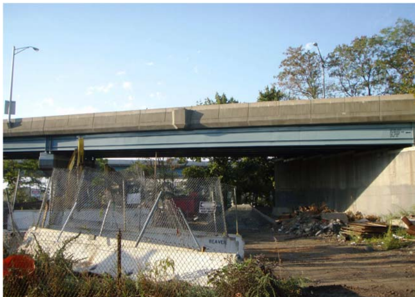
Figure 5: Structure No. 1913154 (Cherry Weber & Associates, PC, 2010)
