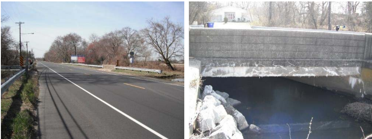
Figure 5: Overview of Structure 0118150 – US206 over Cedar Branch
