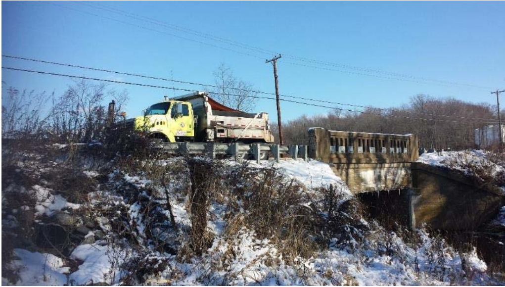
Figure 32: Truckload Test on Structure 1703152
