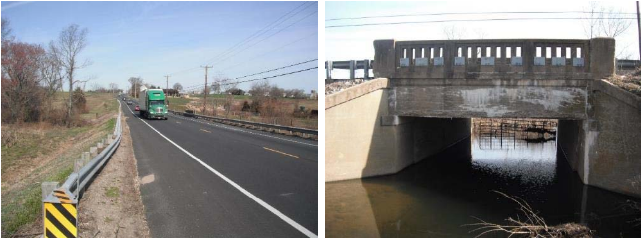
Figure 24: Overview of Structure 1703152 – US40 over Salem Creek
