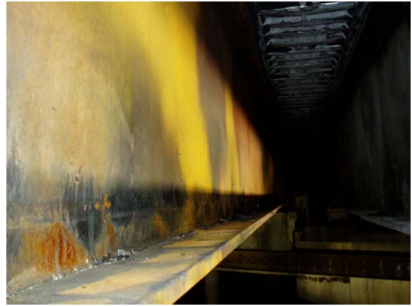
b. Debris on Flanges
