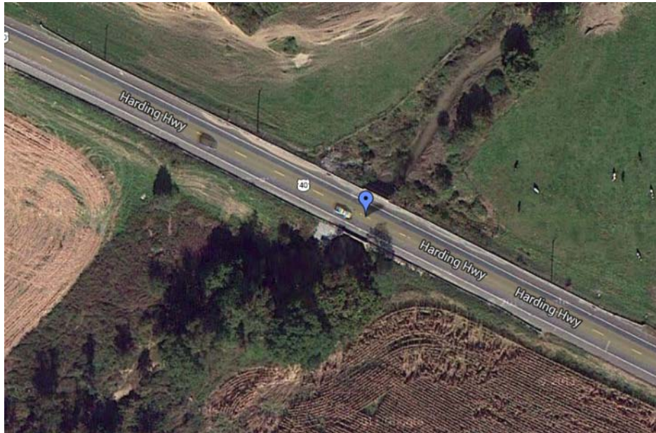
Figure 25: Structure 1703152 – Aerial View
