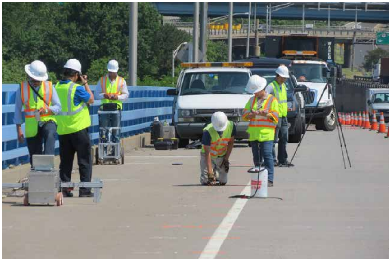
Figure 1. NDE surveys on Route 9 southbound bridge deck.
