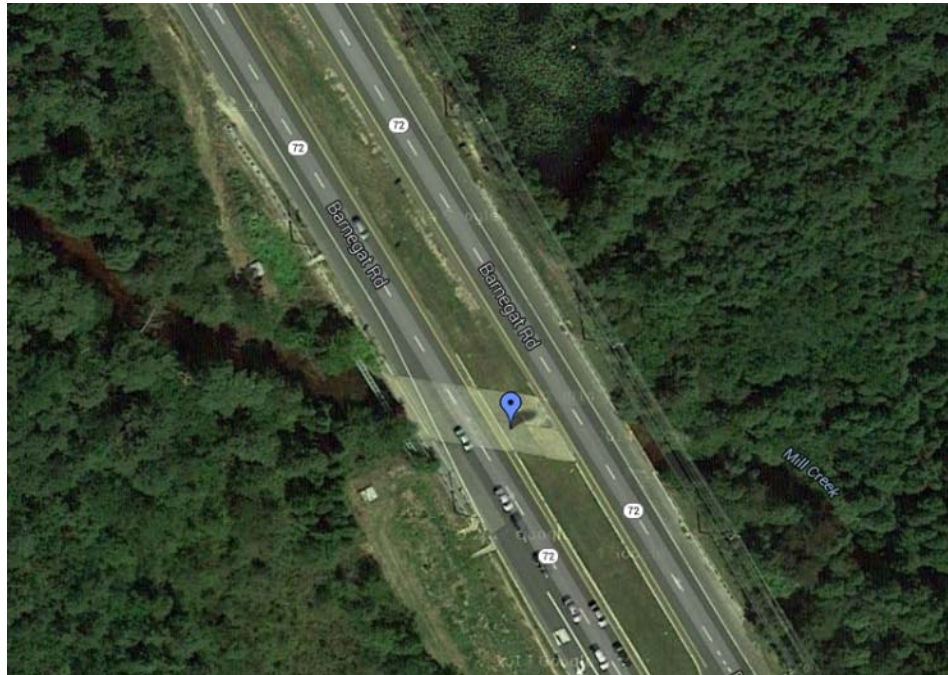
Figure 38: Structure 1512152 – Aerial View
