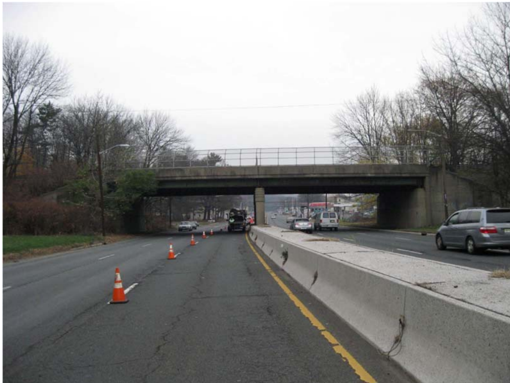
Figure 11: Structure No. 2003150 (Stantec Consulting Services, 2009)
