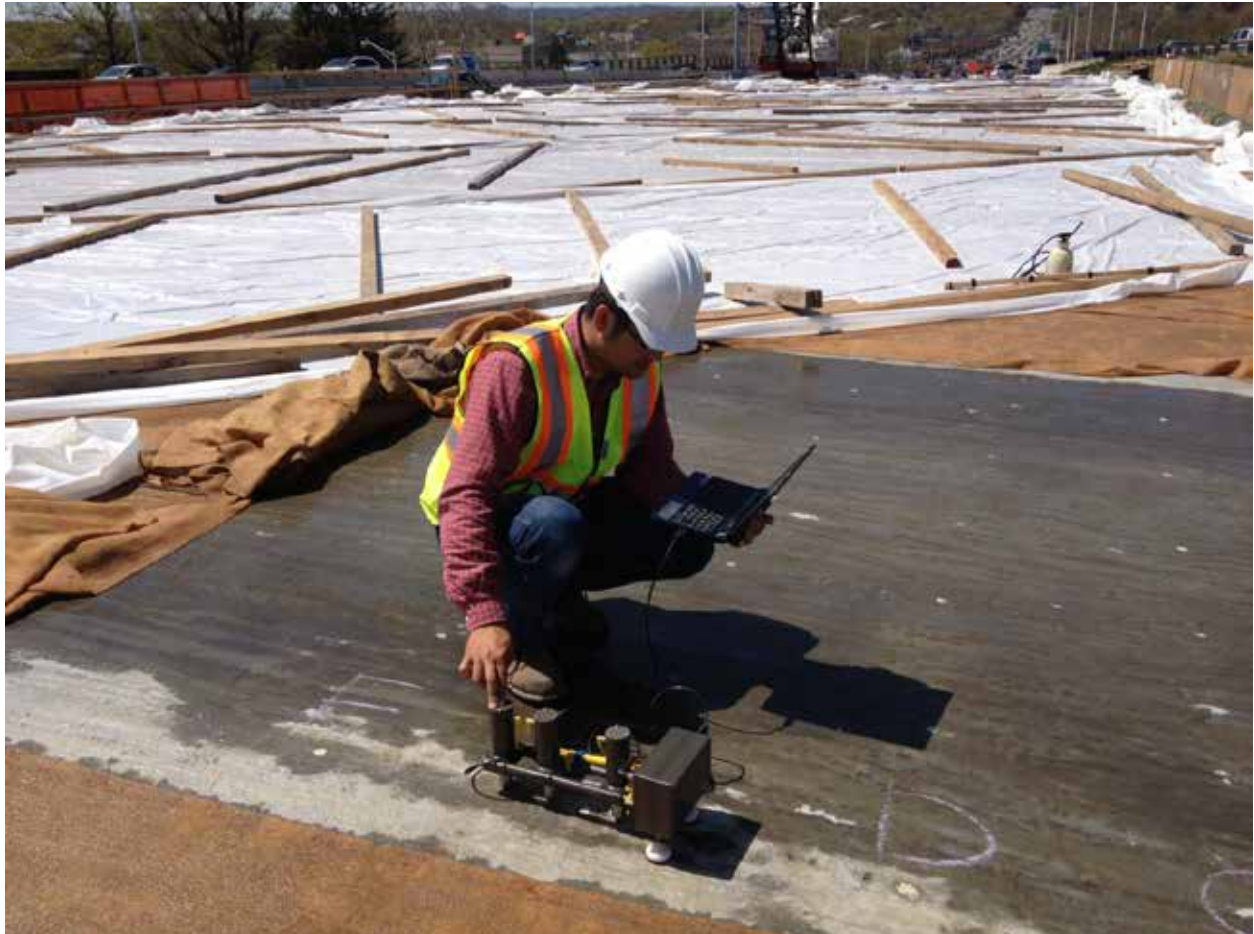
Figure 1. Concrete modulus measurement on Route 3 over Passaic River bridge (June 11, 2013).
