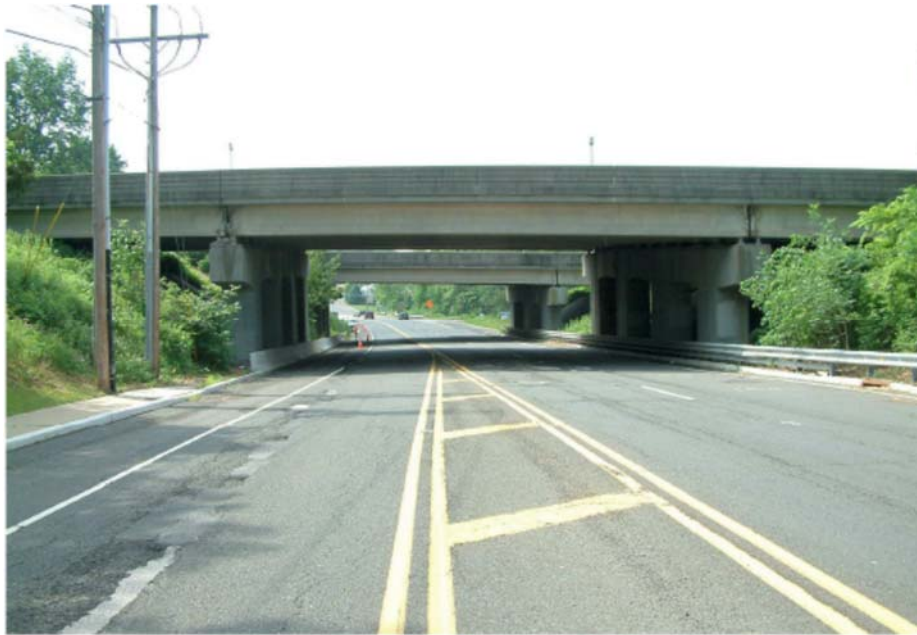
Figure 7: Structure No. 1817156 (Management, 2011)
