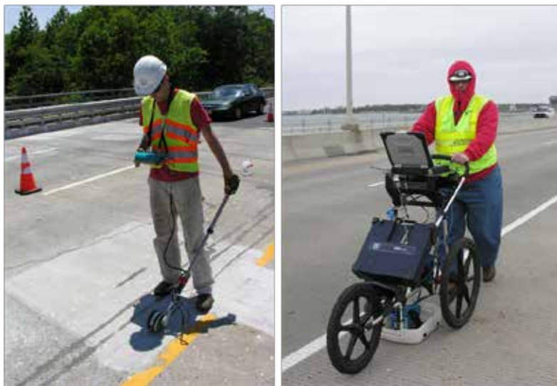
Figure 3 - Corrosion activity assessment using HCP (left) and GPR survey (right).
