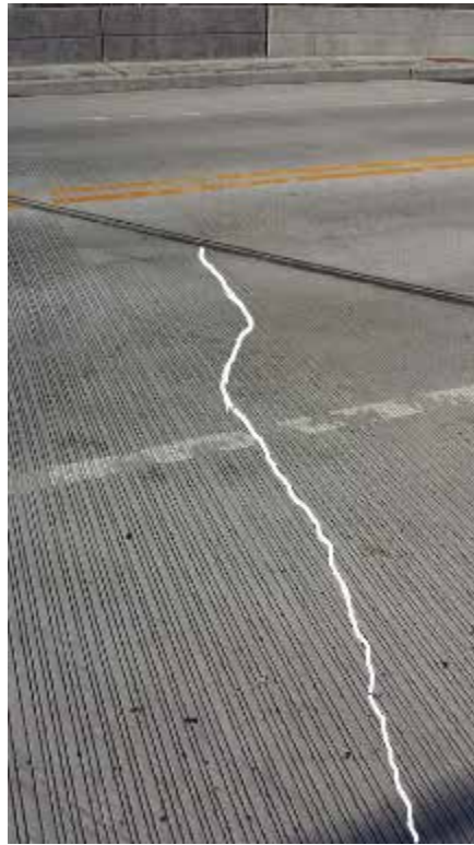
Figure 32: Collings Ave Bridge Deck Cracking – Acute Corner
