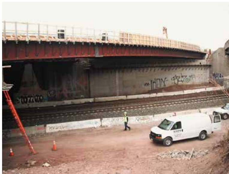
Figure 2: ROUTE 3 Passaic River Crossing
