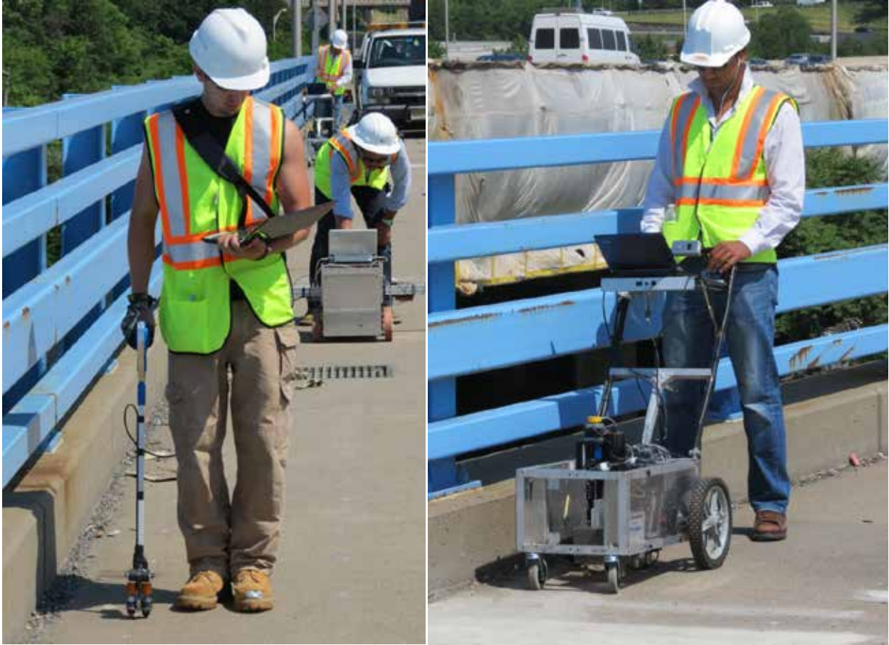
Figure 2. IE "Cane" (left) and PSPA testing (right) on Route 9 southbound bridge.
