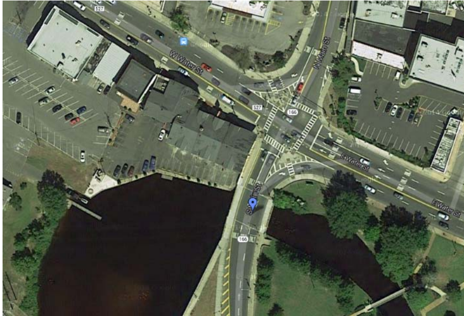
Figure 45: Structure 1516152 – Aerial View
