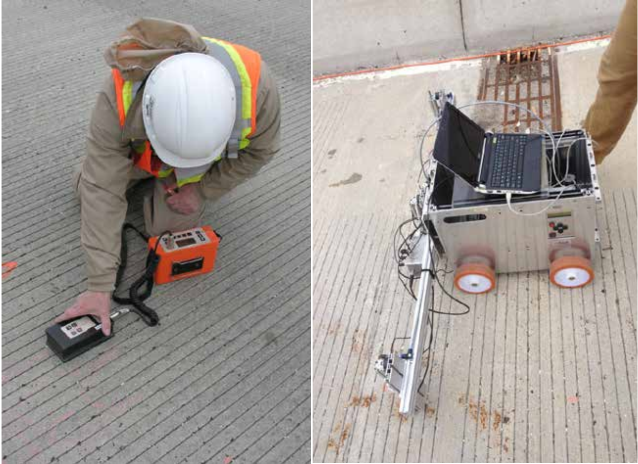
Figure 2. Pachometer measurement to identify a rebar location for half-cell potential probe connection (left) and IE testing using Stepper (right) on Route 52 bridge.
