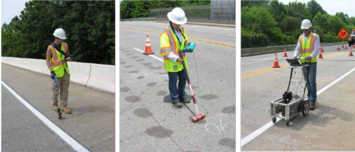
Figure 2 - Delamination detection using IE (left), assessment of corrosive environment using ER (middle), and concrete quality assessment using USW (right).
