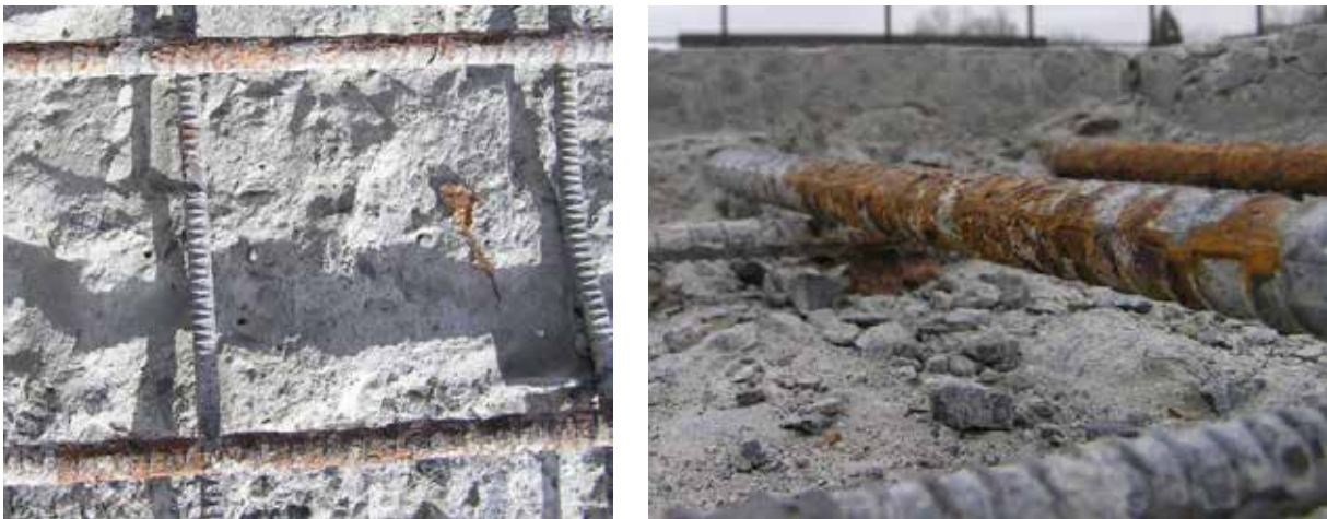
Figure A1. Rebar corrosion.
