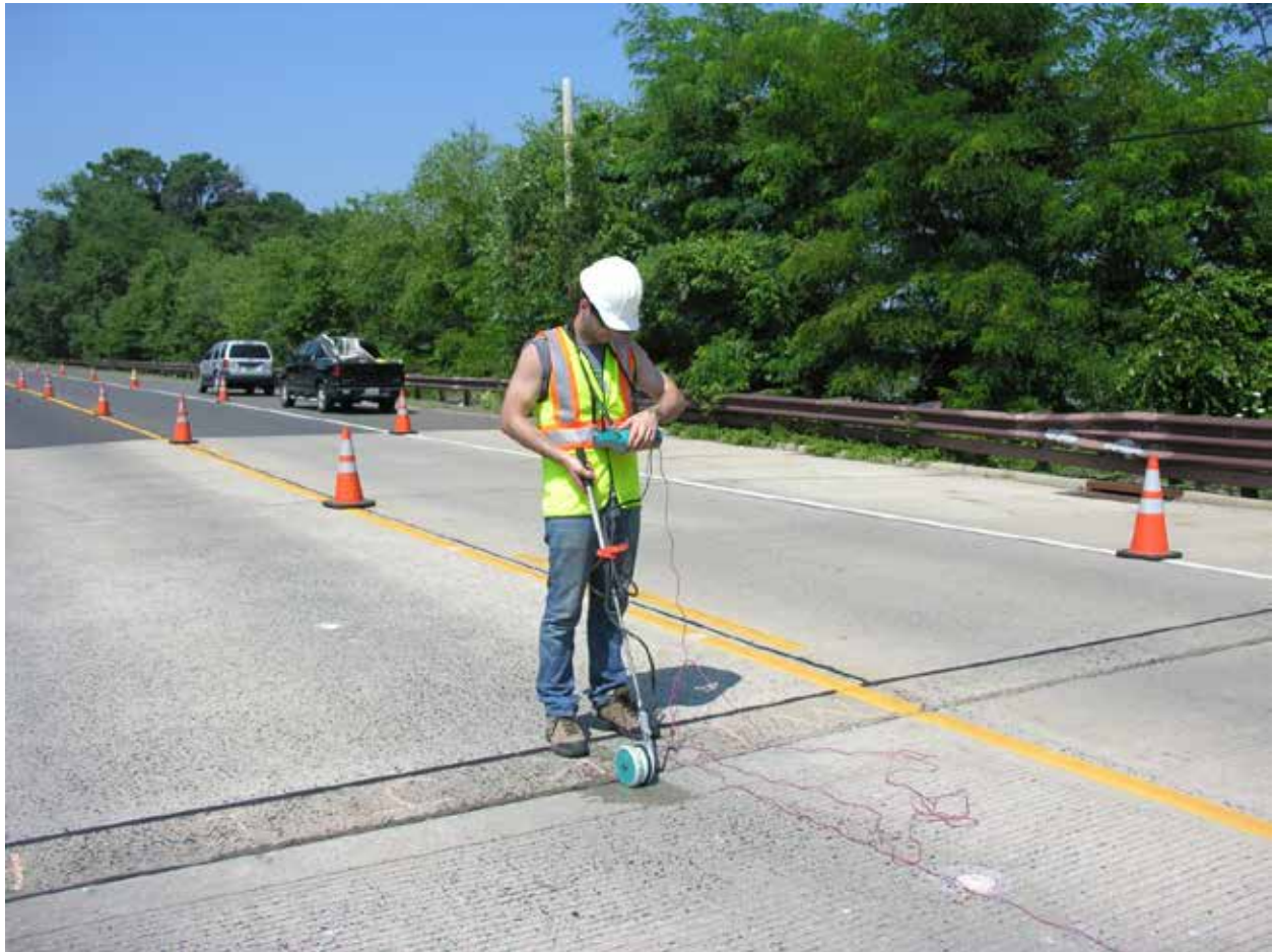
Figure 1. Half-Cell Potential measurement on the Route 70 over Biphams Creek Bridge.
