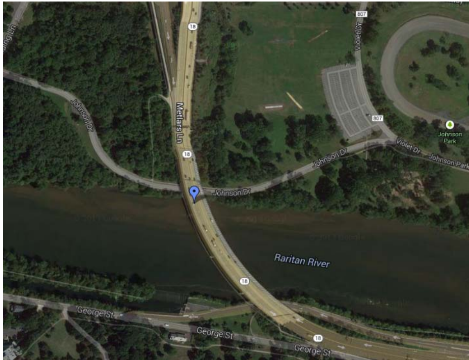
Figure 59: Structure 1237155 – Aerial View
