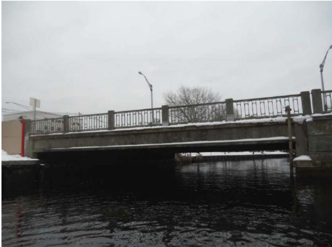
Figure 9: Structure No. 1516152 (LS Engineering Associates Corporation, 2010)
