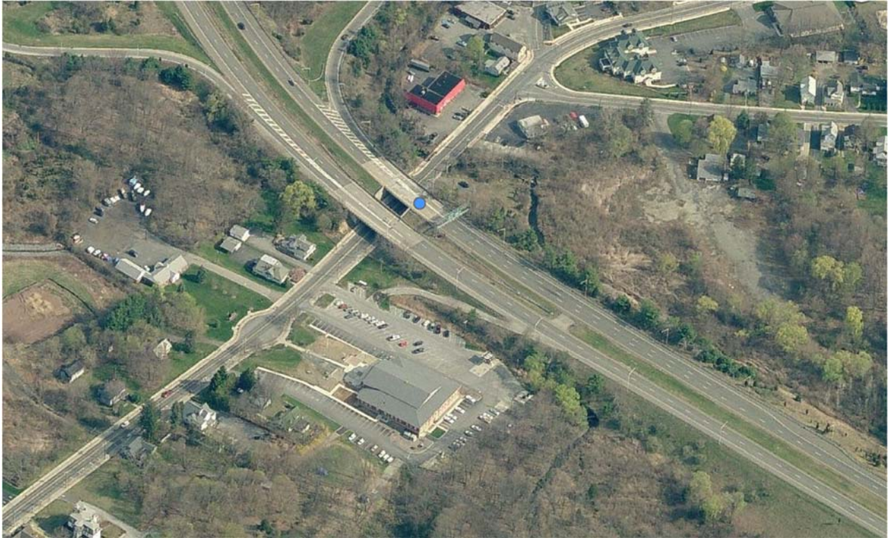
Figure 6: Structure No. 1913154 Aerial View
