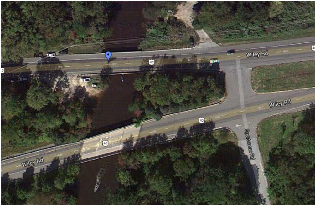
Figure 69: Structure 1701151– Aerial View
