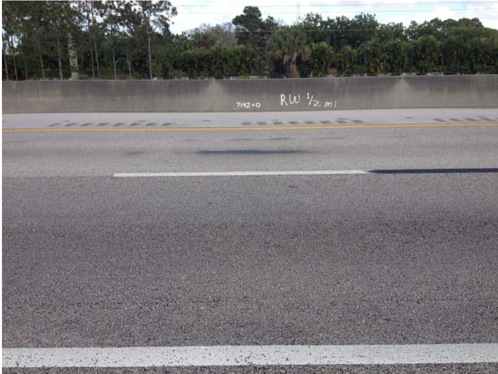
Figure 3.24 - Flushed Area on Florida Turnpike near MP 133
