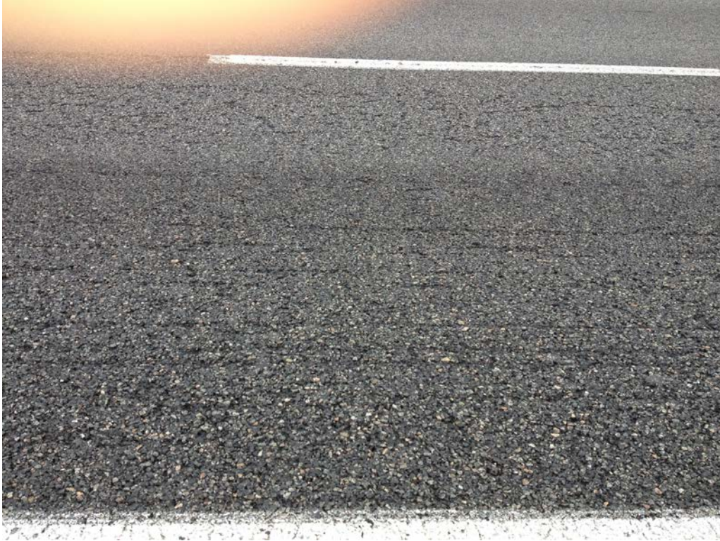
Figure 3.17 - Raveling on I-75 in Hamilton County (MP 461-462)
