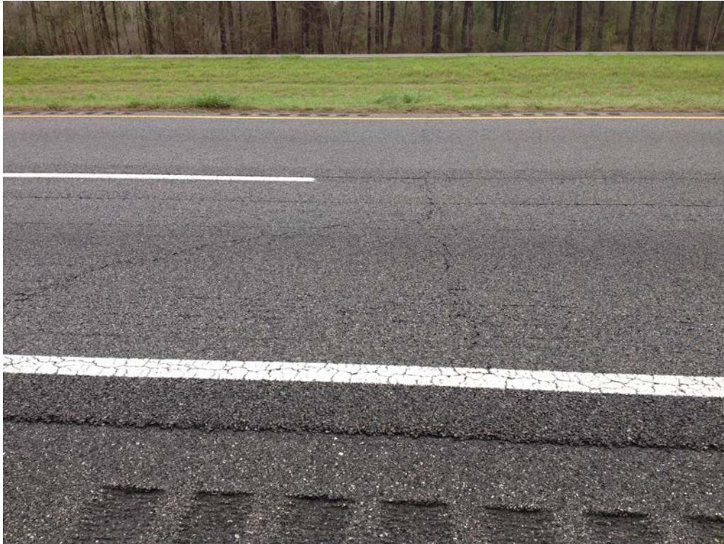
Figure 3.20 - Transverse Cracking on I-10 (MP 229-230)
