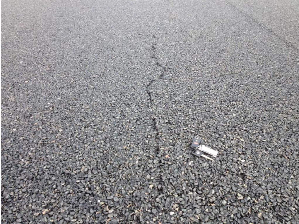
Figure 3.15 - Longitudinal Crack on SR-20
