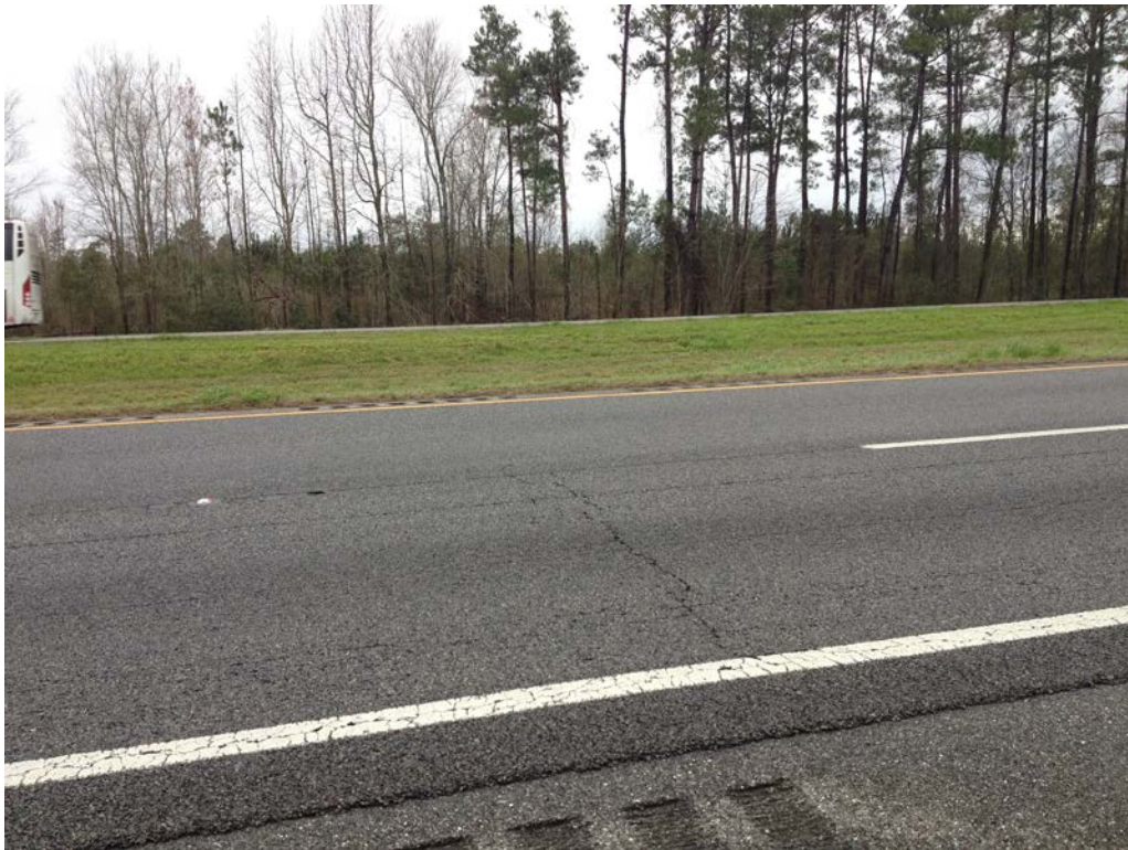
Figure 3.19 - Transverse Crack on I-10 (MP 229-230)
