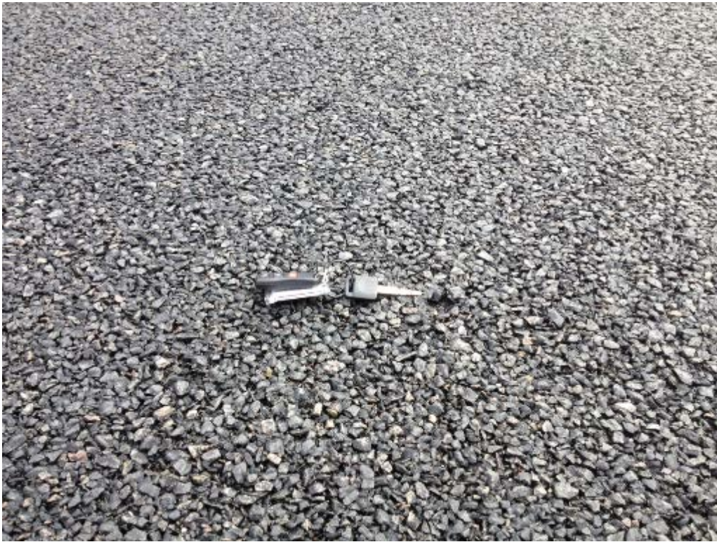
Figure 3.14 - Aggregate Pop-out on SR-20
