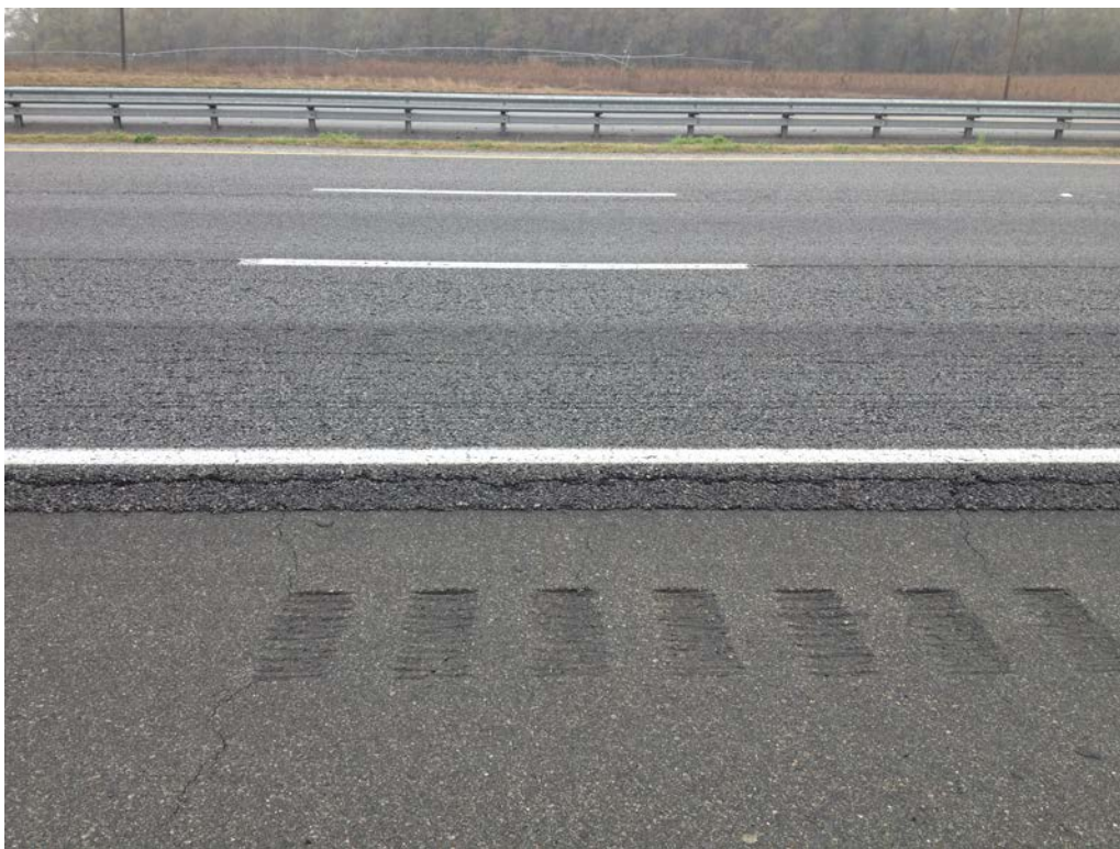
Figure 3.16 - Rutting on I-75 in Hamilton County (MP461-462)
