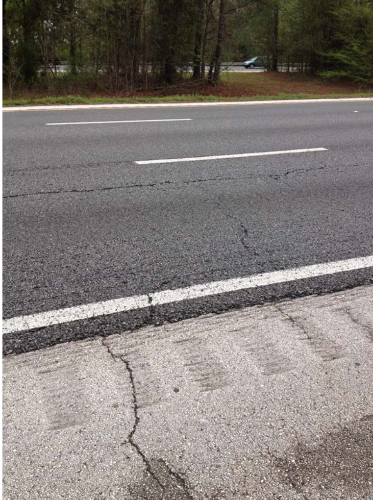
Figure 3.23 - Transverse Crack on I-75 in Marion County
