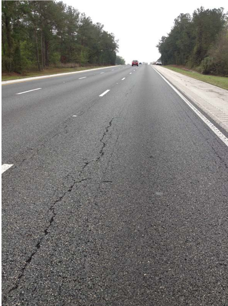
Figure 3.21 - Longitudinal Crack on I-75 in Marion County
