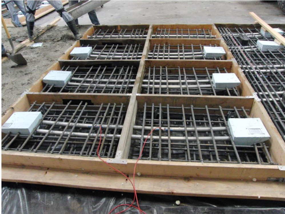
Figure 12: Small Specimens Prior to Concrete Placement.
