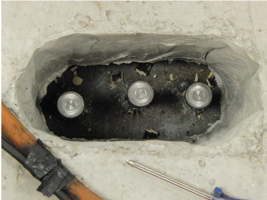
Figure 21: Shear Studs After Welding.
