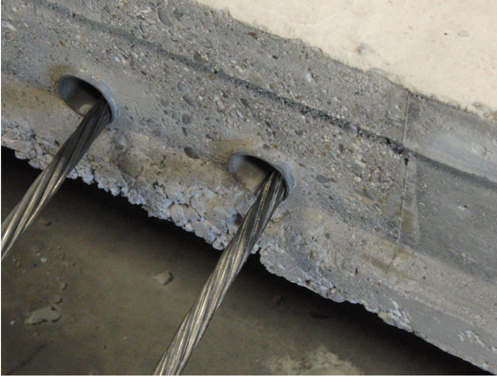
Figure 15: Aggregate Exposed in Joint for Grouting.
