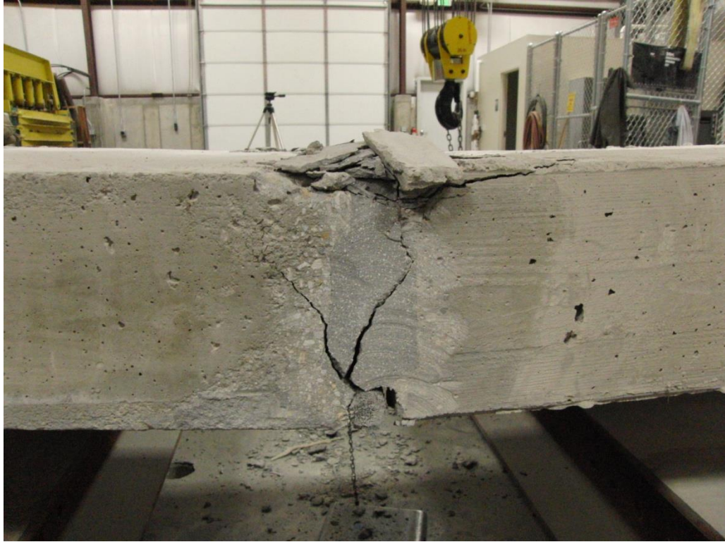
Figure 23: Flexural Failure of Small Scale Specimen.
