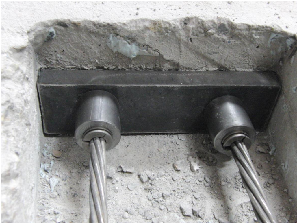
Figure 17: Post-Tensioning Bearing Plate and Connection.
