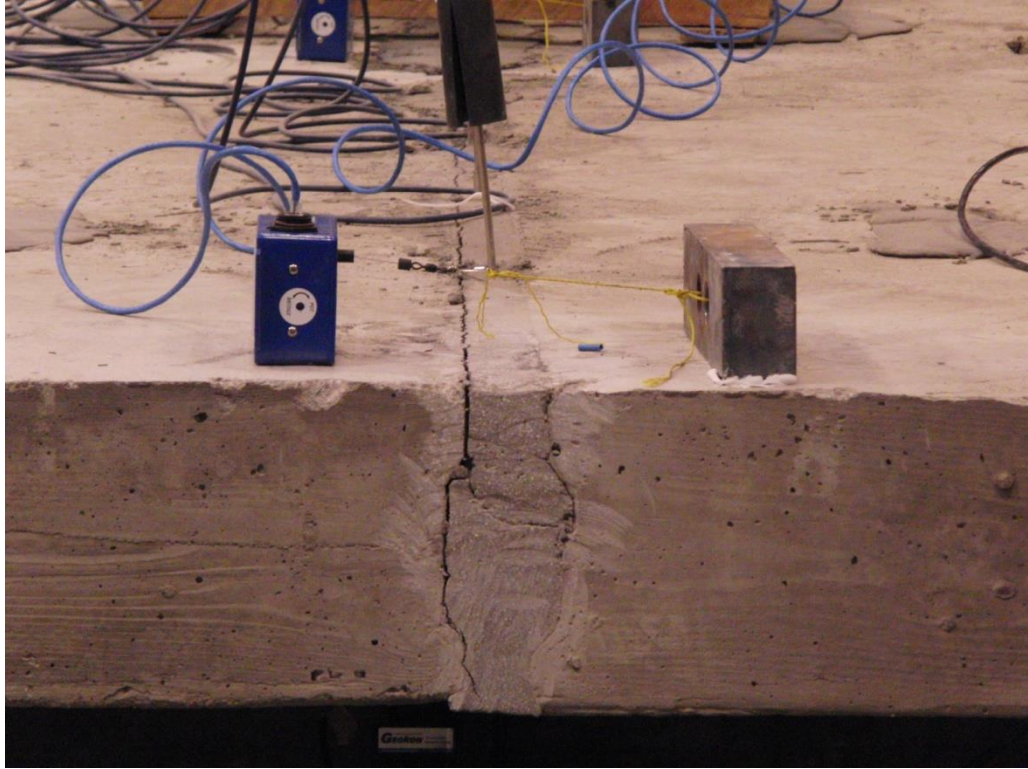
Figure 30: Cracking Along Joint.
