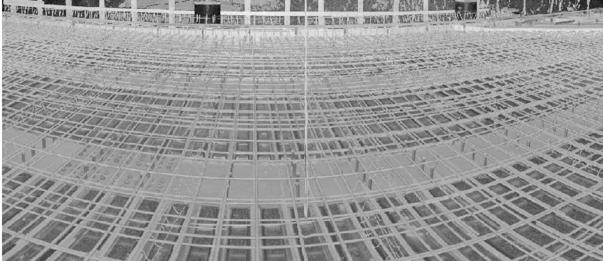
Figure 21 Bridge deck rebar in 3D point cloud
