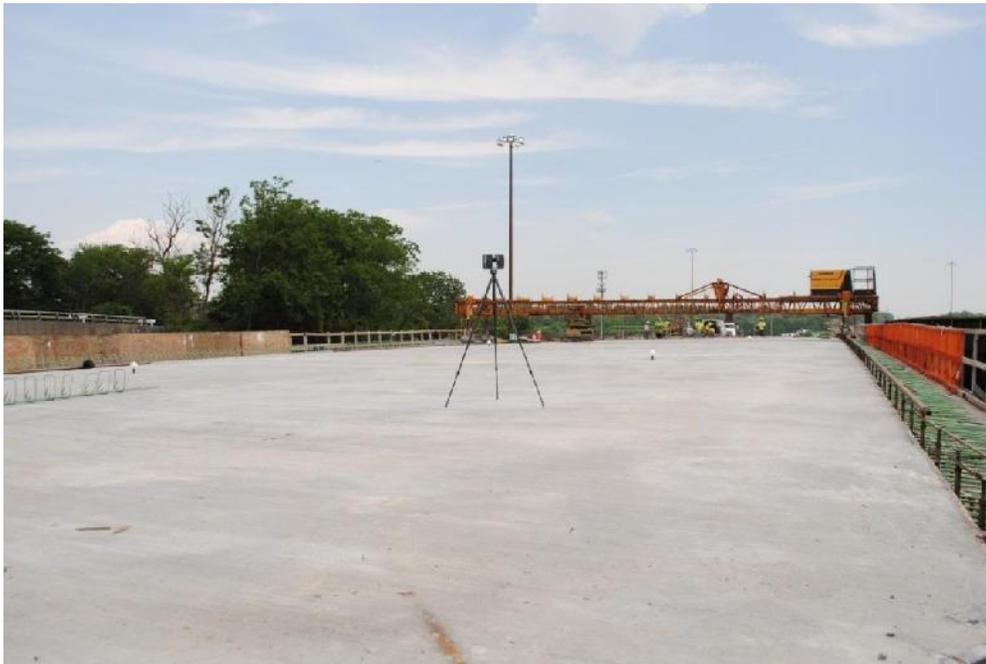
**Figure 17 Scanning the concrete surface**
