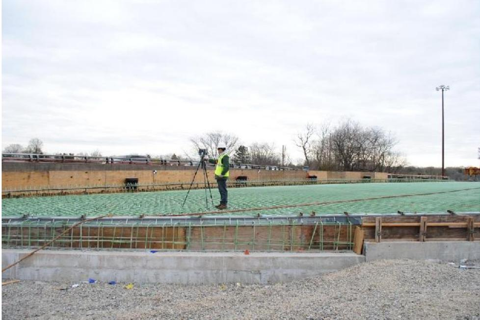
Figure 14 Scanning the rebar surface
