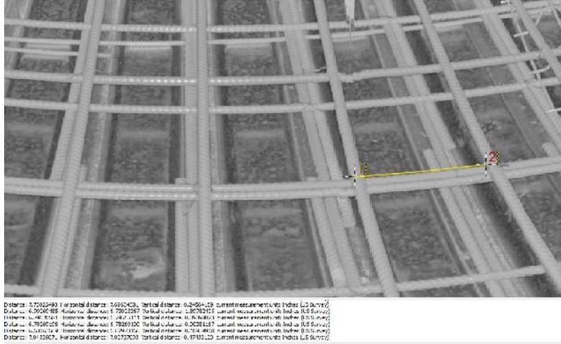
Figure 23 Spacing of top transverse rebar
