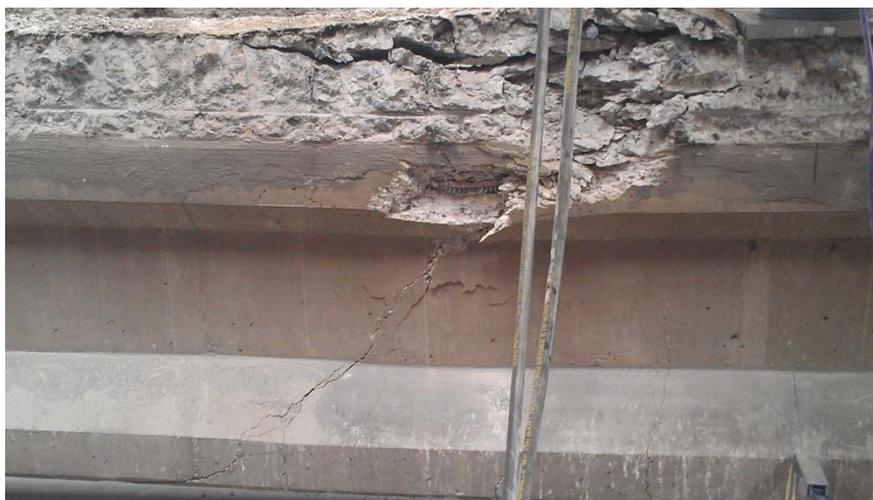
Figure 29 Shear failure in G1-2d(a)
