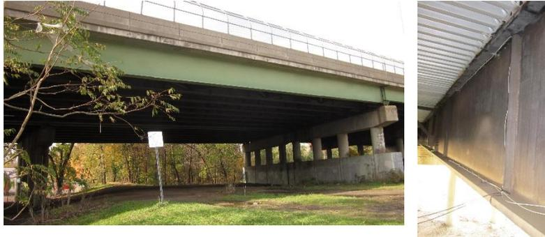
Figure 4. Left: The US202/NJ23 overpass consisting of concrete slab supported on steel girders. Right: Detail of the sensor positioning at the top and the bottom [6].
