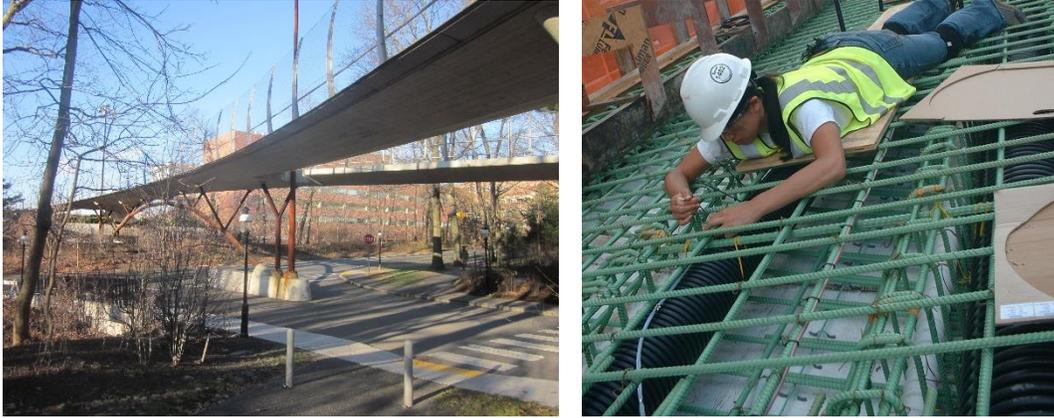
Figure 6. Left: View to the Streicker Bridge. Right: Embedding sensors in the Streicker Bridge.
