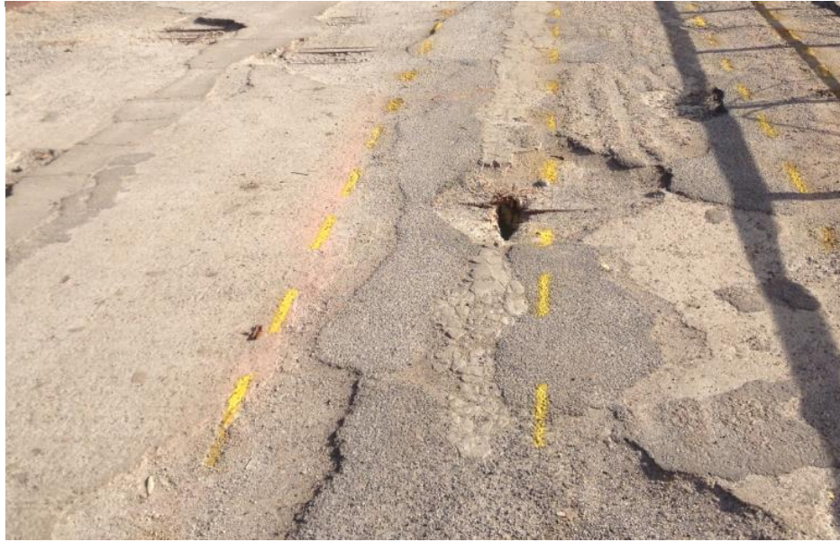
Figure 2.6 Damaged superstructure deck surface
