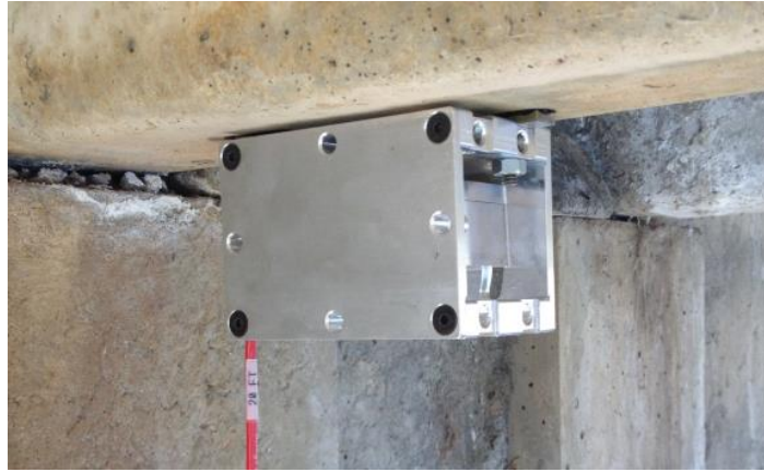
Figure 2.14 Tiltmeter installed at the bridge abutment.
