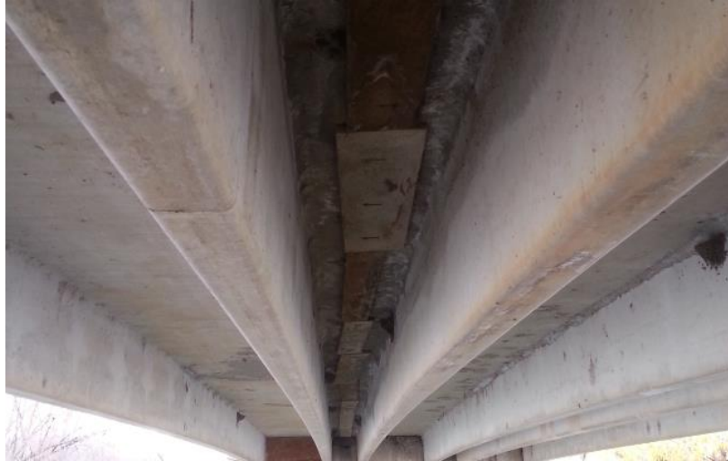
Figure 2.7 Girders showing no cracking
