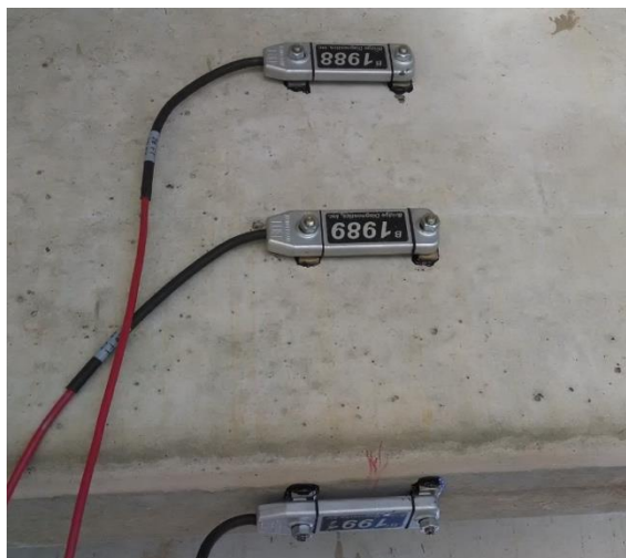
Figure 2.13 Strain gages installed on double tee girder stem
