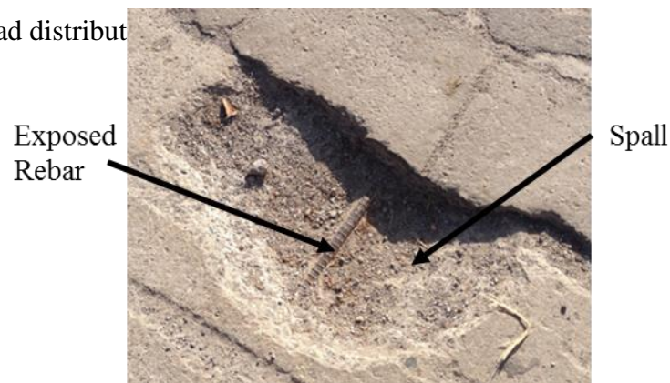
Figure 2.5 Pothole on the bridge superstructure structural deck component
