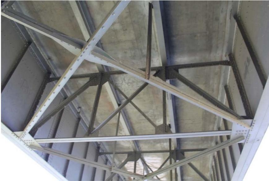
*Figure 3.12 Picture of Vertical and Transverse Diaphragms Members*
