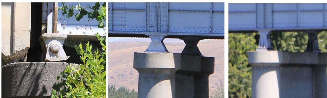
Figure 3.5 Pictures of Roller, Pinned, and Roller in Fixed Shoe Bearings
