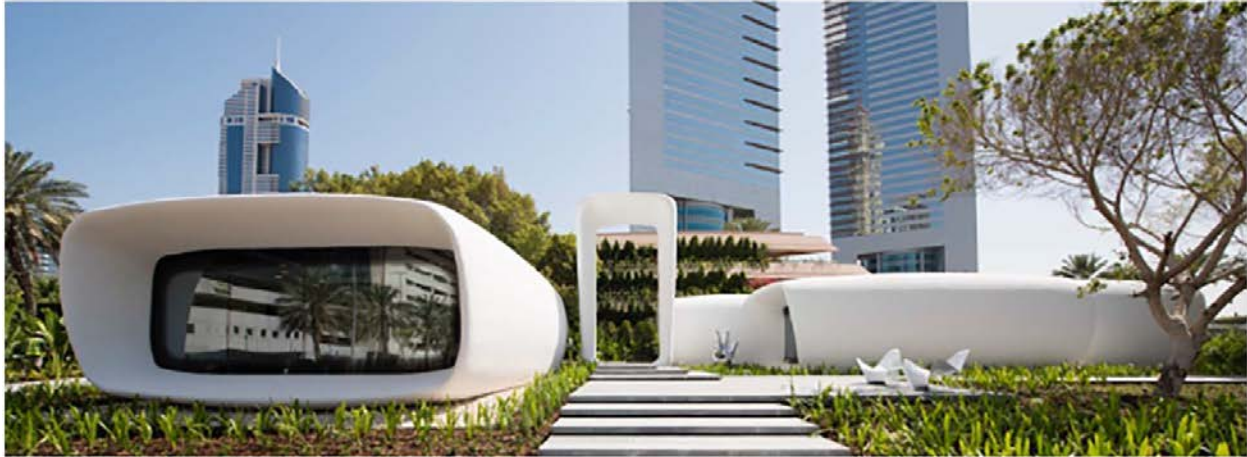
Figure 15 3D printed office of the future in Dubai (Killa Architectural Design 2016).
