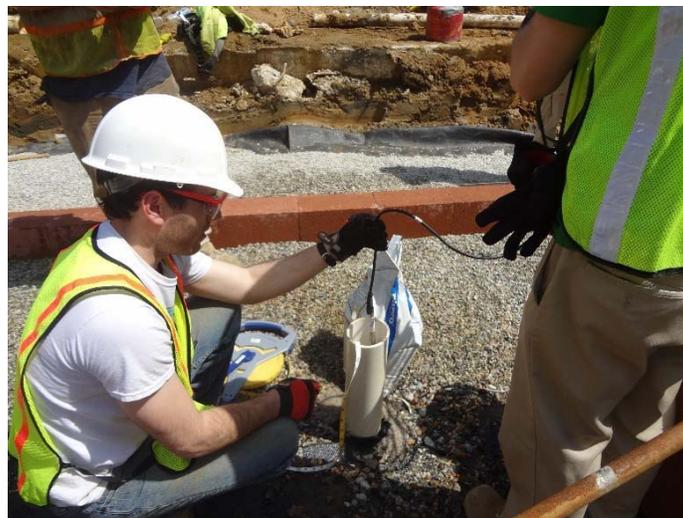
**Figure 3.5 Piezometer sensor installation**
