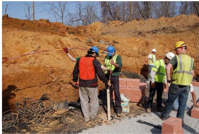
**Figure 3.3 IPI sensor array installation**
