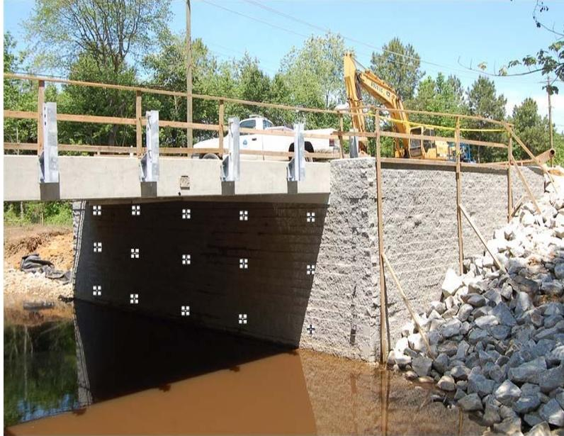
**Figure 3.14 East abutment facing wall surveying points**
