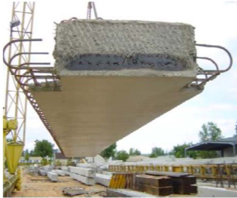
Figure 1-1: Poutre-Dalle system (Bell, 2006)
