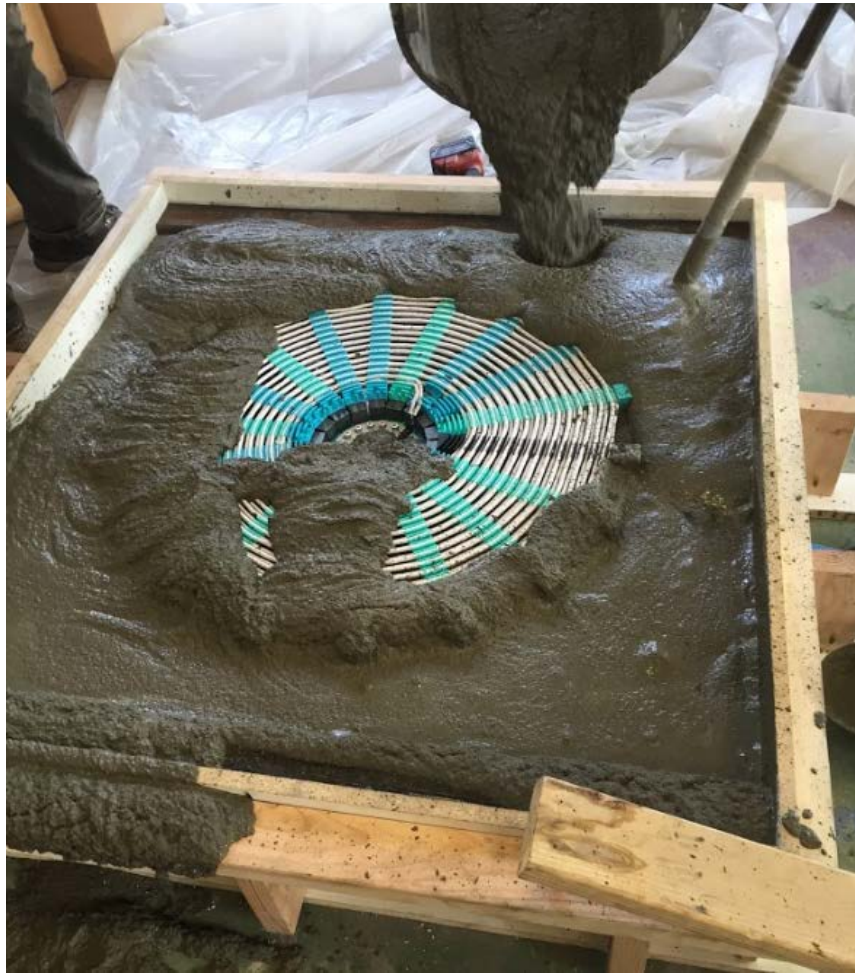
Figure 2.14 Pouring first inductor pad
