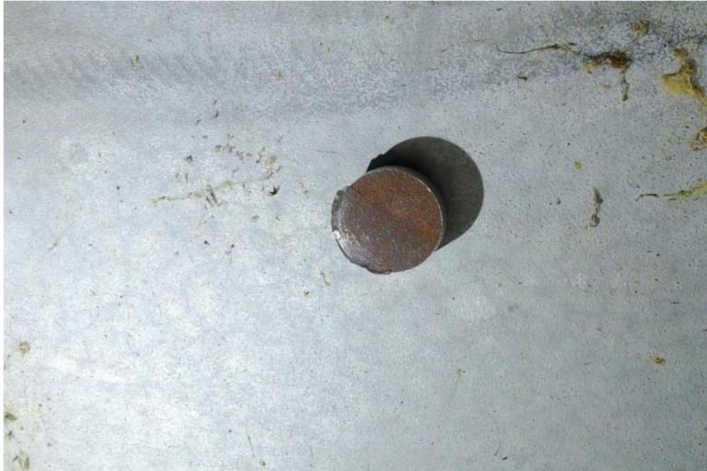
Figure 4.16 Photo of the Test-Piece Taken by DJI Mavic, UWRL Bridge, Bright Condition, Normal Camera Angle, E012
