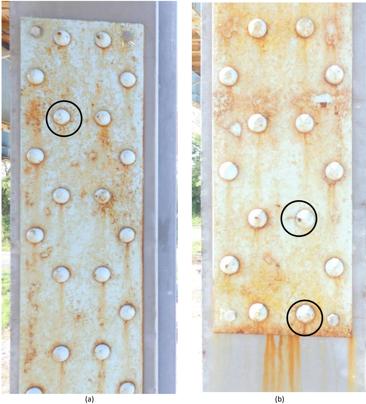
Figure 6.26 Images of the riveted cover plate specimen (a) reported crack on row 3 and (b) reported cracks on row 25 and 27
