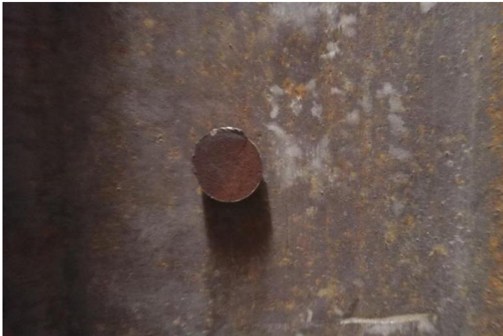
Figure 4.17 Photo of the Test-Piece Taken by DJI Mavic, UWRL Bridge, Dark Condition, Normal Camera Angle, E012
