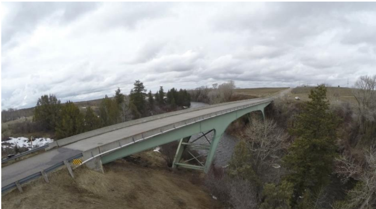
Figure 5.5 Northern Girder of the Fall River Bridge.
