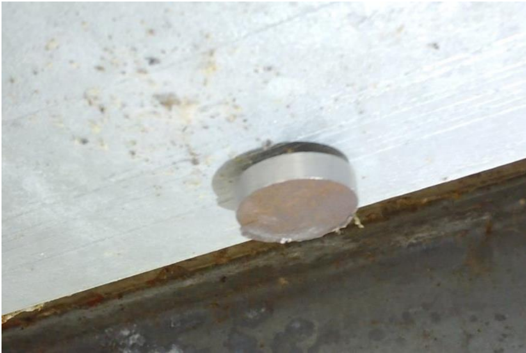
Figure 4.18 Photo of the Test-Piece Taken by DJI Mavic, UWRL Bridge, Bright Condition, Oblique Camera Angle, E012
