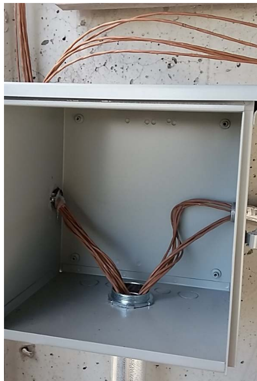
Figure 3.13 West column junction box
