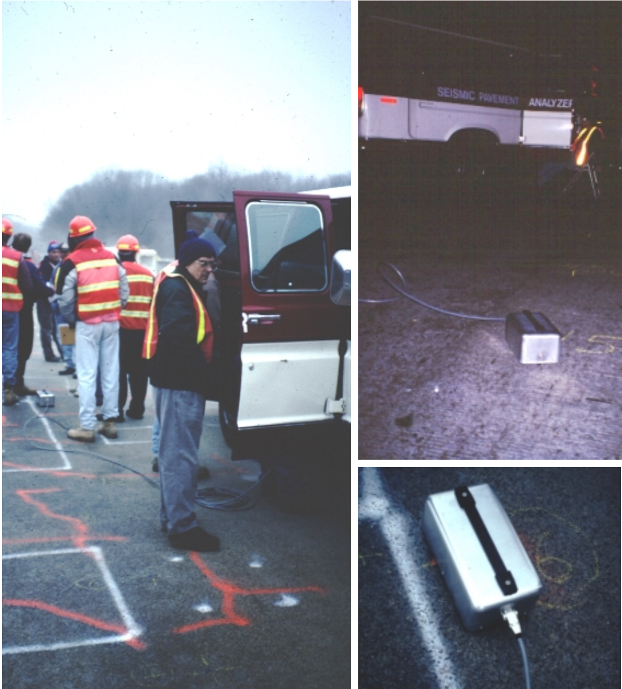
Figure 4.2. Evaluation of bridge decks by PSA.
