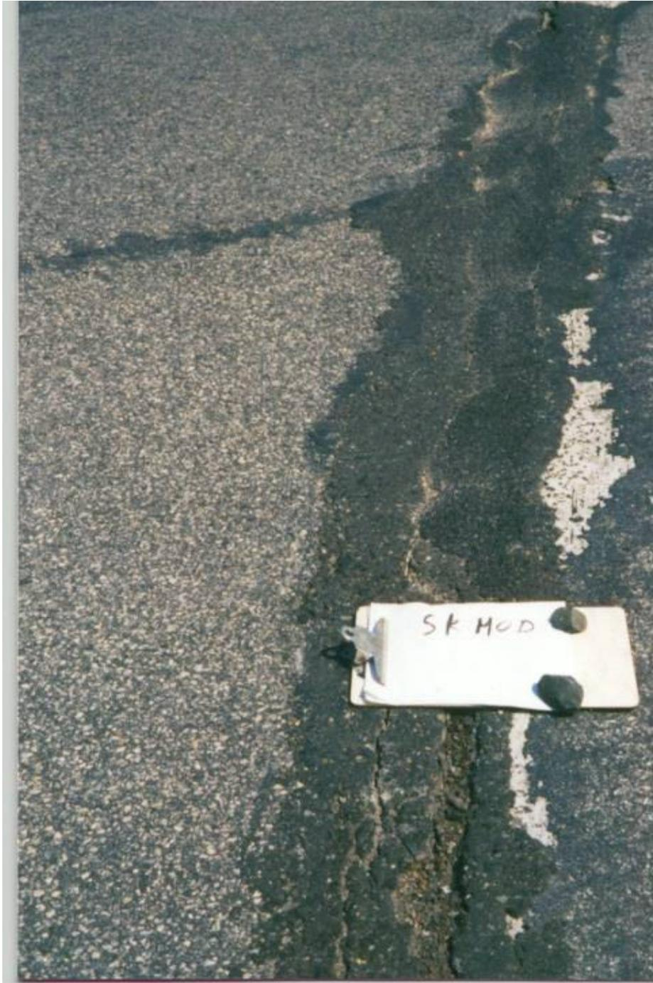
**Figure 48. SuitKote 6 Month Inspection, Rt. 3 WB Ramp to Rt. 21 NB Clifton**
