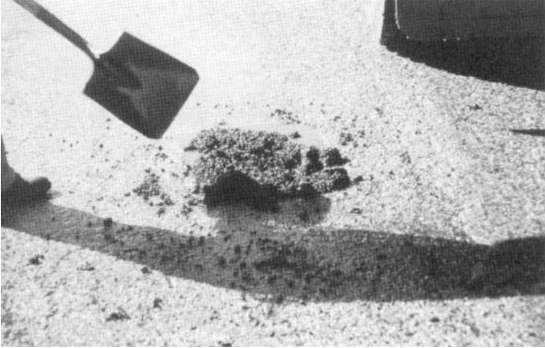
**Figure 6. Throw-and-Roll Repair Method: Placement of Material** <sup>(5)</sup>
