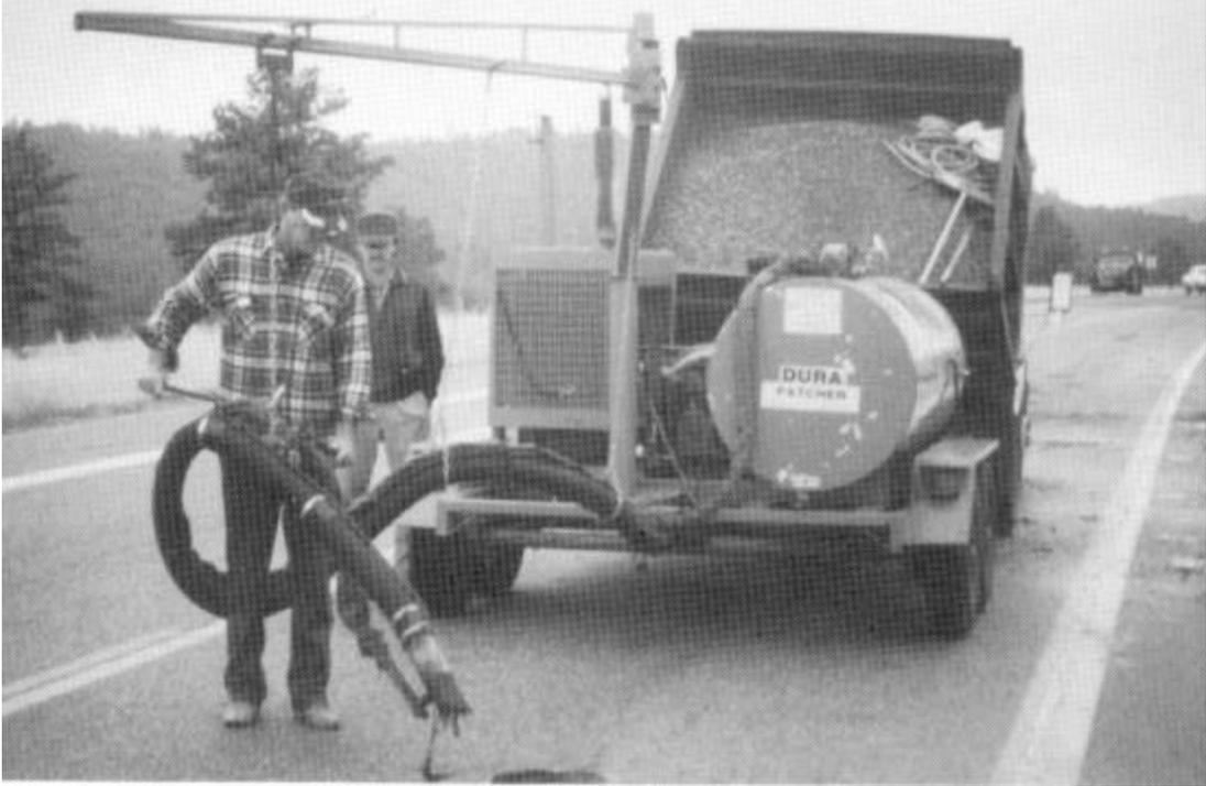
**Figure 10. Spray Injection Method of Pothole Repair <sup>(5)</sup>**
