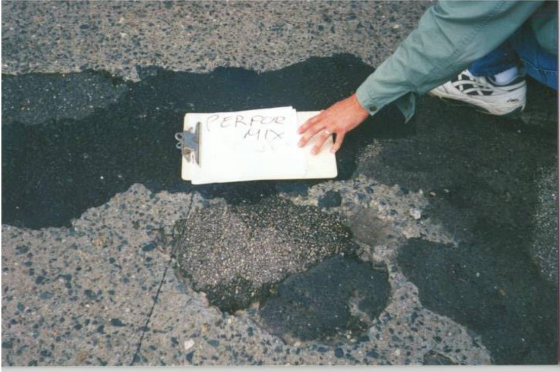
**Figure 40. Performix 6 Month Inspection, Rt. 21 SB MP 11.8 Passaic**
