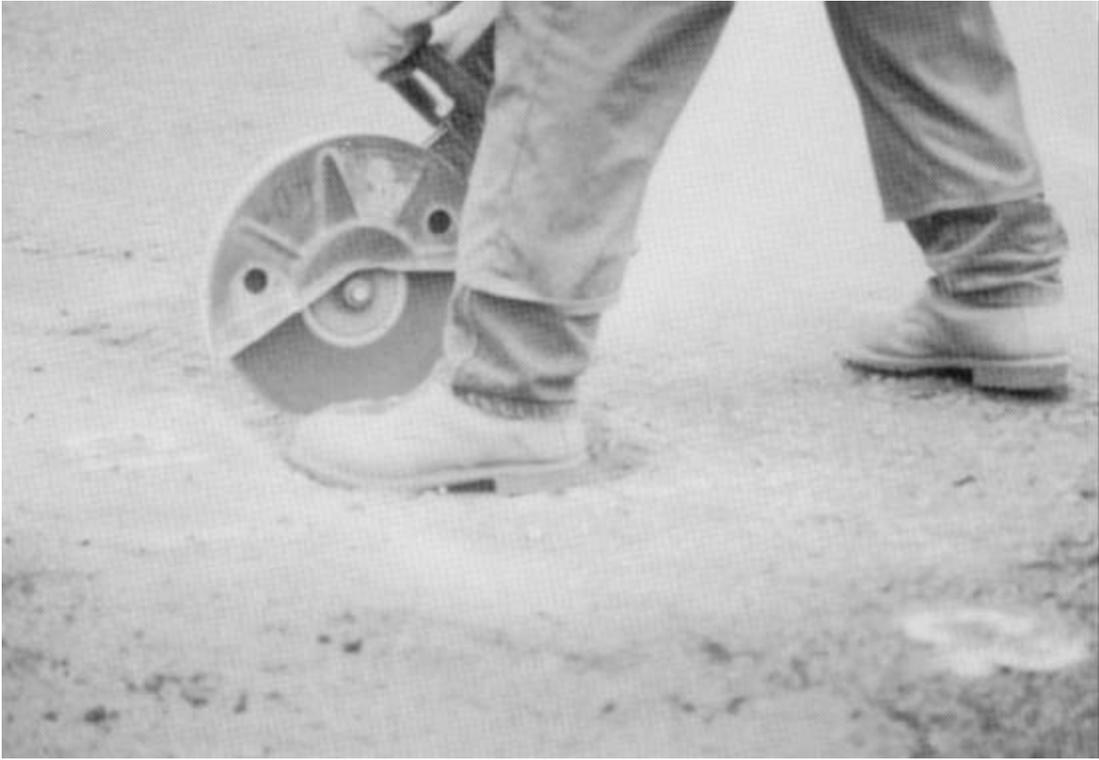
**Figure 8. Semi-permanent Method of Pothole Repair: Saw-Cutting of Edges** <sup>(5)</sup>
