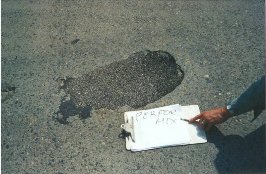
**Figure 41. Performix 6 Month Inspection, Rt. 21 SB 11.8 Passaic**
