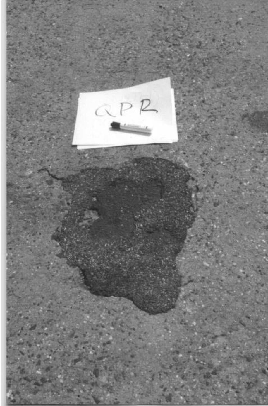
**Figure 46. QPR 6 Month Inspection, Rt. 21 SB MP 12.0 Passaic**
