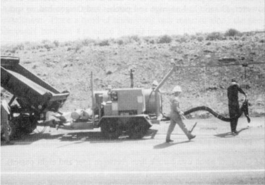
**Figure 11. Spray Injection Method of Pothole Repair <sup>(5)</sup>**
