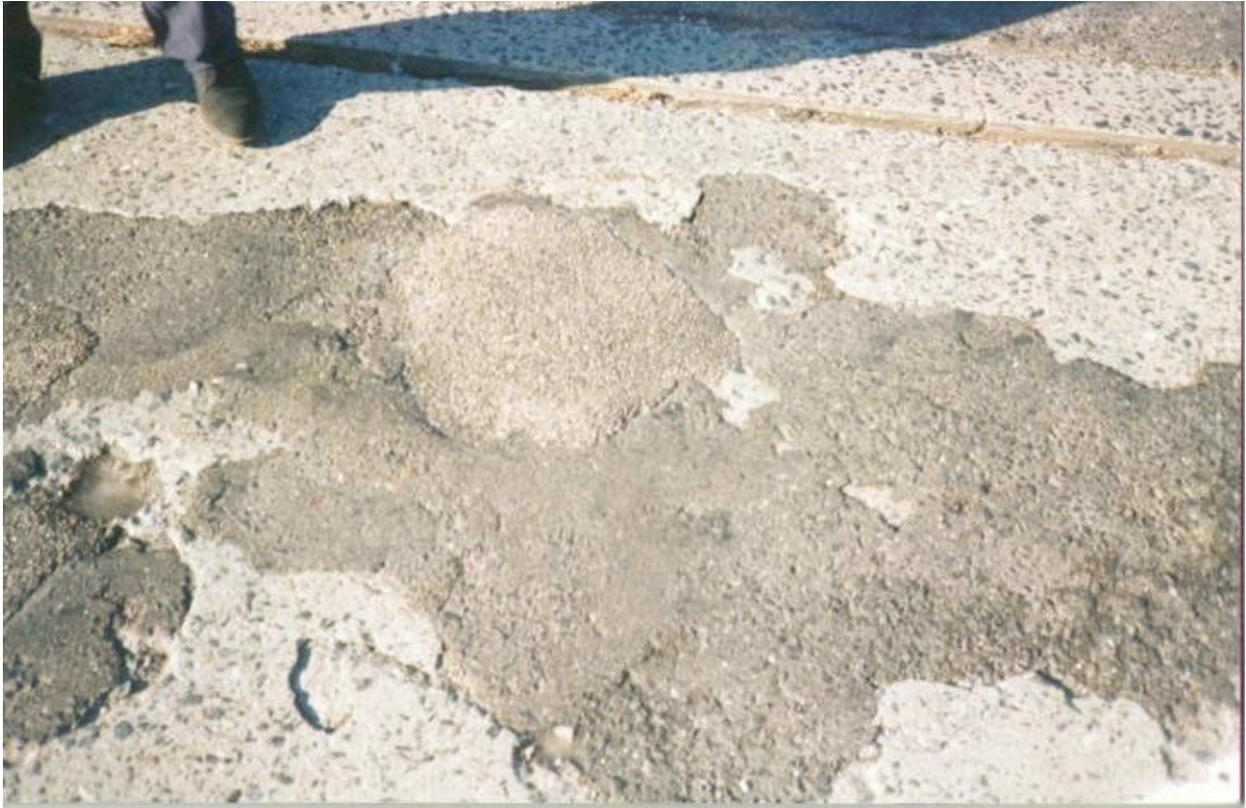
**Figure 38. Performix- 2 Month Inspection, Rt. 21 SB MP 11.8 Passaic**
