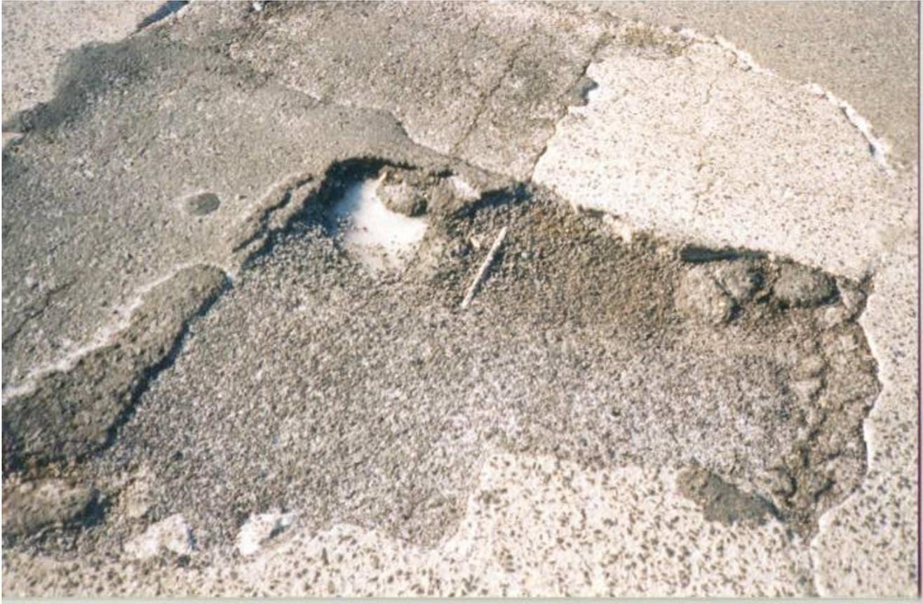
**Figure 42. Permapatch 2 Month Inspection, #1 Rt. 21 NB Passaic,
