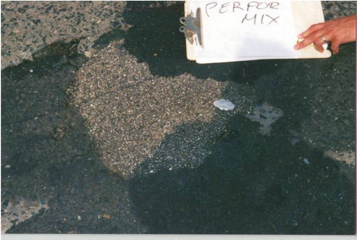
**Figure 39. Performix 6 Month Inspection, Rt. 21 SB MP 11.8 Passaic**
