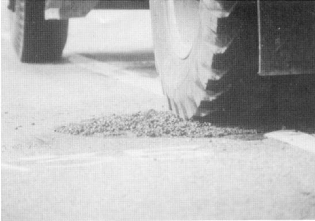
**Figure 7. Throw-and-Roll Repair Method: Compaction of Material Using the Wheels of a Truck on Site<sup>(5)</sup>**
