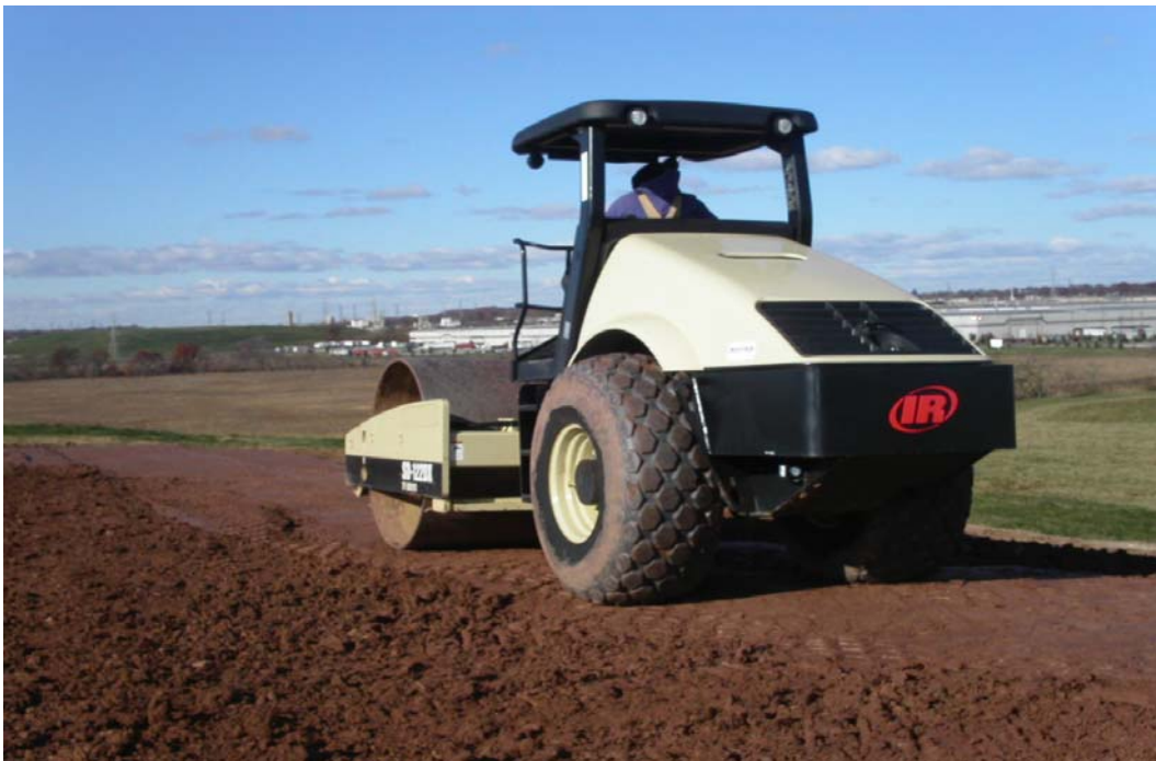
Photo #12. Compaction of the Red Clay at the ILR Landfill
