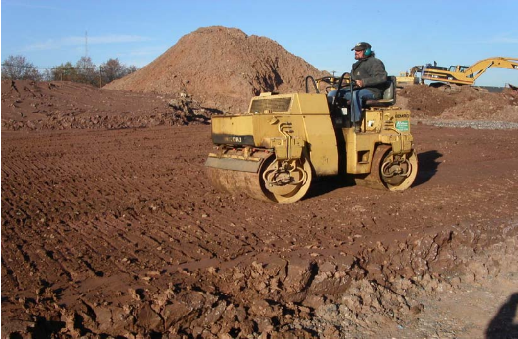
Photo #7. Compaction of the Red Clay
