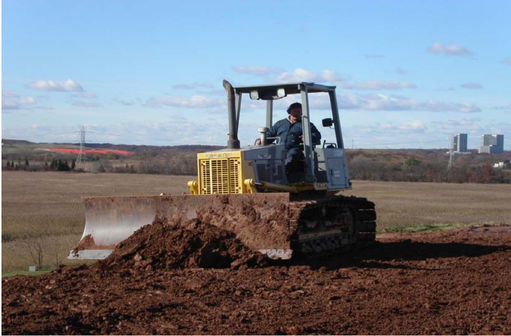
Photo #11. Spreading of the Red Clay in 6-inch Layers at the ILR Landfill
