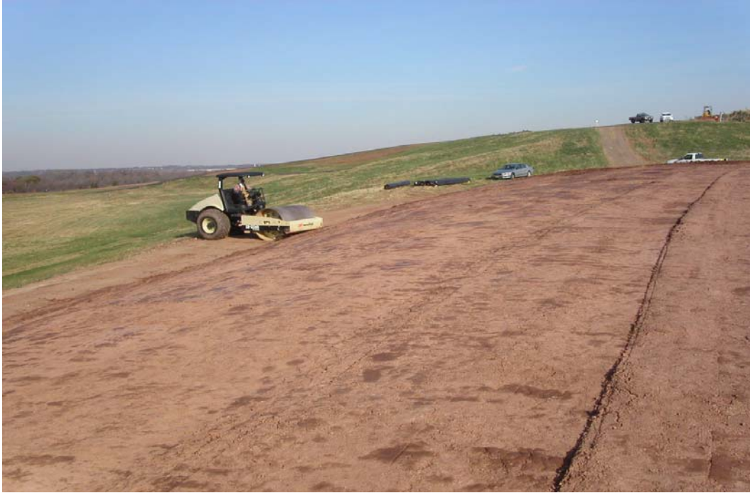
Photo #13. Compacted Red Clay
