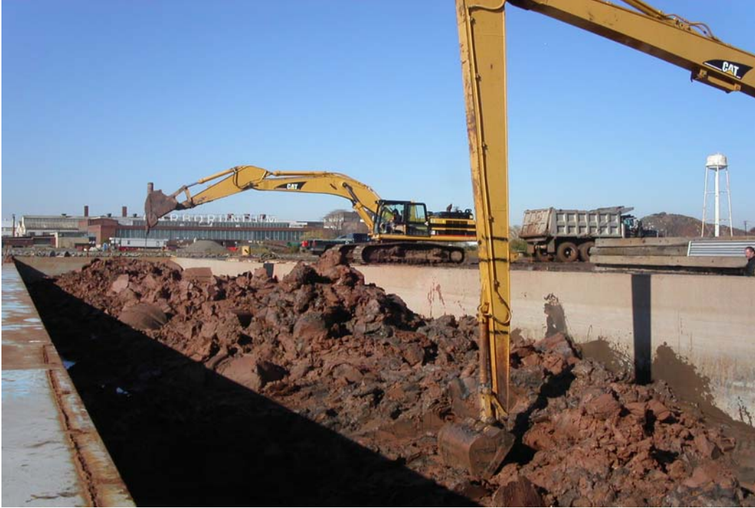
Photo #3. Unloading of the Red Clay
