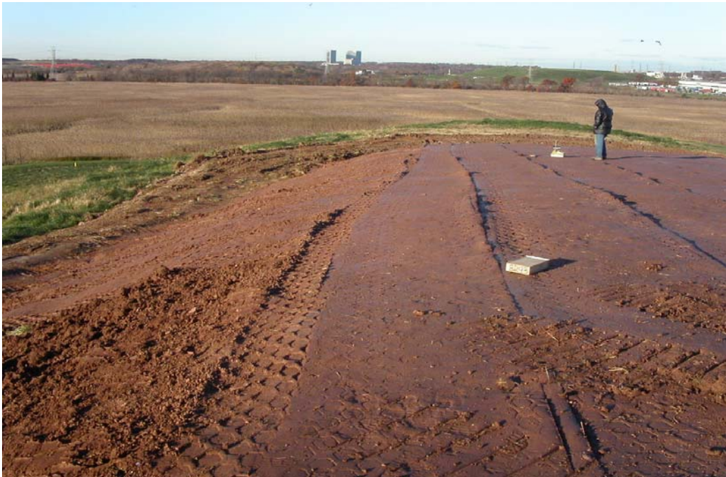
Photo #14. In-situ Density Testing of the Red Clay
