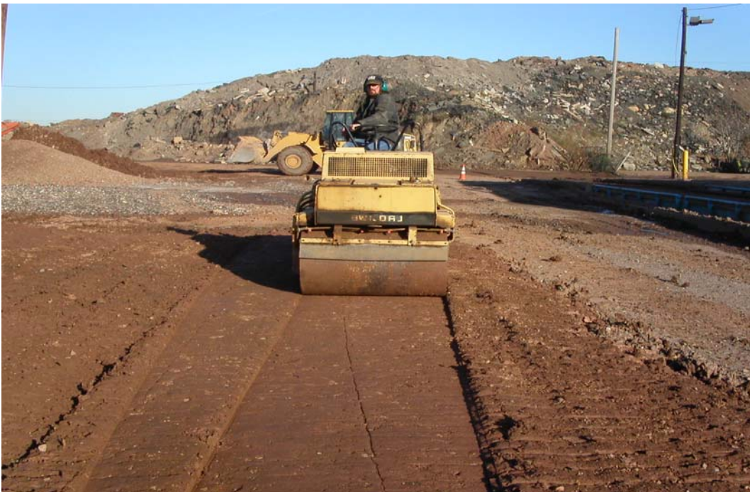
Photo #8. Compaction of the Red Clay
