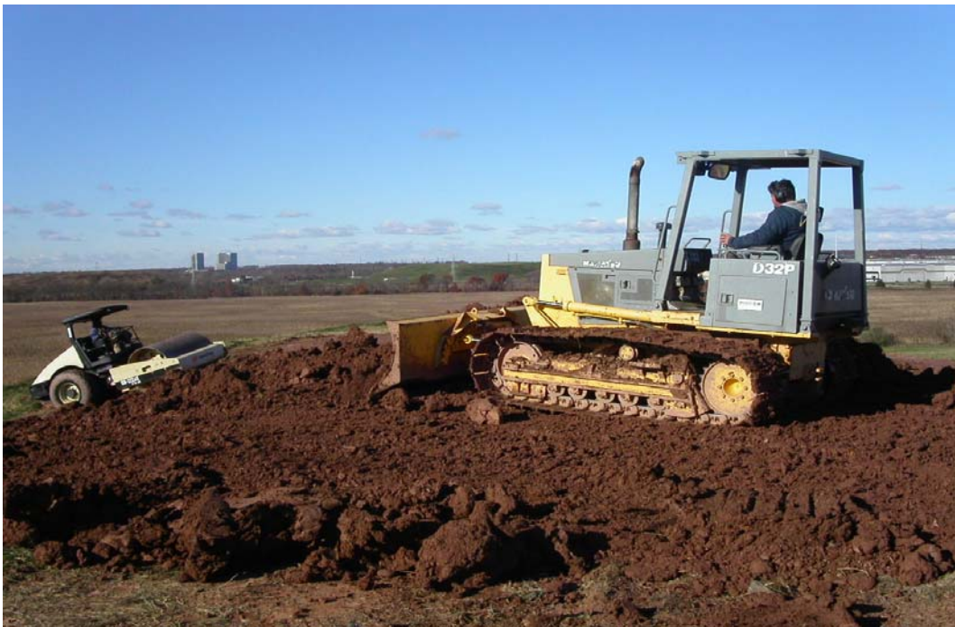
Photo #10. Spreading of the Red Clay in 6-inch Layers at the ILR Landfill
