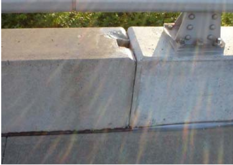
Figure 6. Uncoated Concrete Block Next to a Coated One
