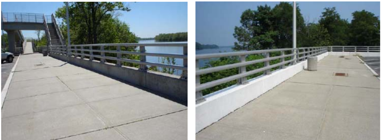
Figure 5. Uncoated Concrete Surface (on the left) and Coated Surface (on the right)
