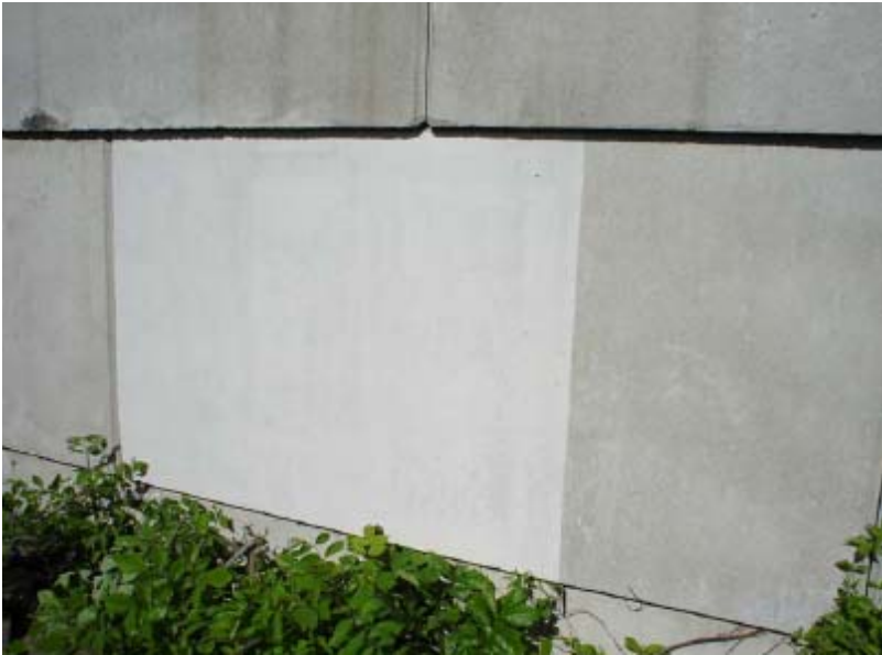
Figure 4. Test Patch (More Than Two Years Old)
