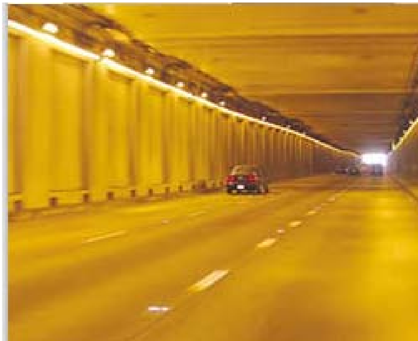
Figure 40 : Tunnel light pipe
