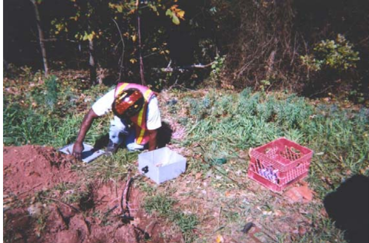
Figure 64 Photograph of control/junction box linked to sensor wires and ready to be buried.
