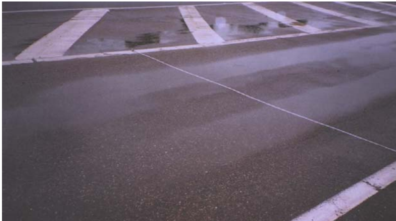
Figure 55 Final proposed location for the installation of the sensor assemblies.
