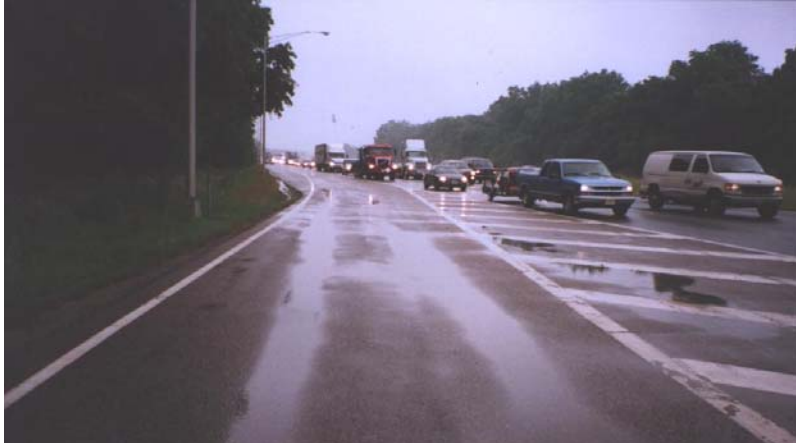
Figure 54 Field observation of water ponding in the wheel paths.
