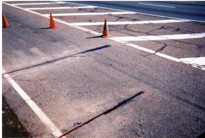
Figure 63 Photograph of the completed WIM installation at the Route 287 weigh station.
