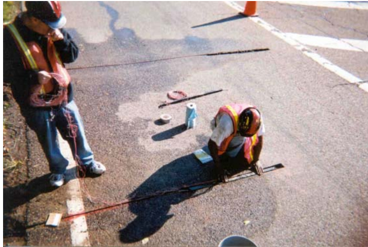
Figure 61 Photograph of ceramic-polymer composite sensor assembly being placed in groove at the Route 287 weigh station.
