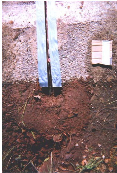
Figure 60 Photograph of the groove with the wires and plastic conduit ready for epoxy infiltration.
