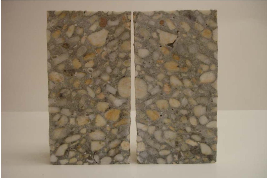
Figure 36 – Cross Sectional View of PCC Core Taken from Rt 34N in New Jersey
