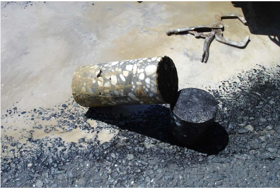
Figure 21 – Extracted Portland Cement Concrete Core from Pre-Overlaid Pavement
