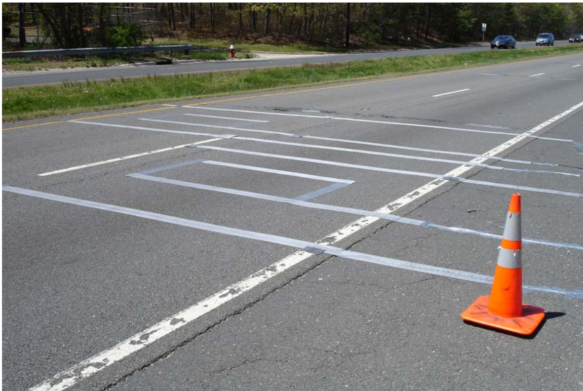
Figure 19 – Weigh-in-Motion/Automated Vehicle Classifiers (WIM/AVC)
