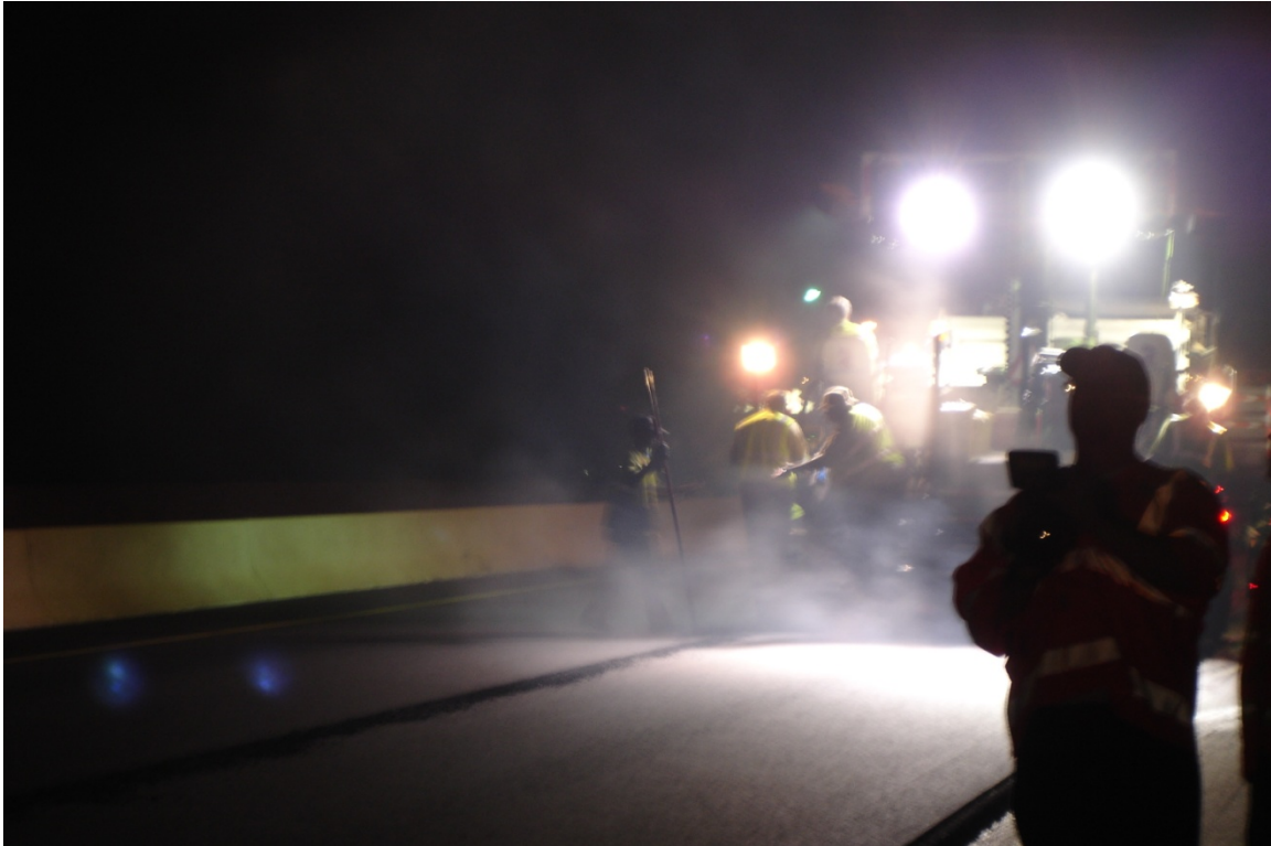
Figure 10. Emissions Behind the Paver on the NJDOT Rt. 38 Warm Mix Project
