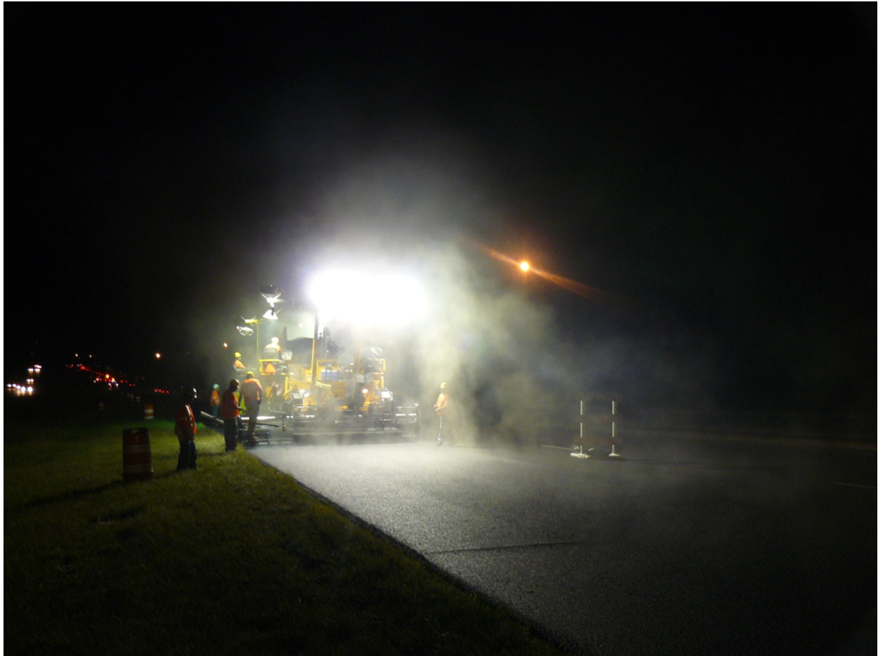
Figure 56. Photo of Emissions Due to Paving an Asphalt Rubber OGFC Mixture
