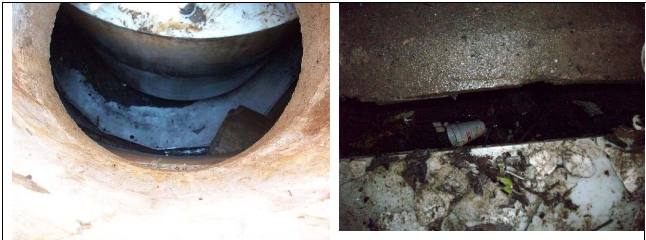
Figure 16. Damaged coupler connecting the device
