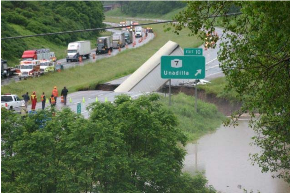
Figure 1. Collapse of a Culvert Crossing I-88 on June 28, 2006
