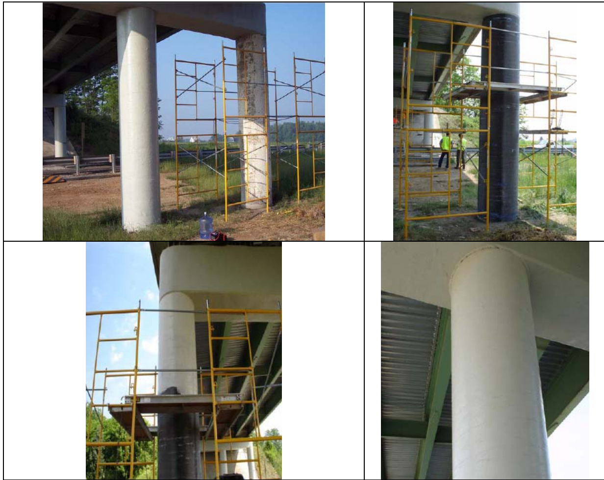
Figure 1 a) Column after cleaning b) Column wrapped with carbon tape c) During final coating application d) Column after final coating
