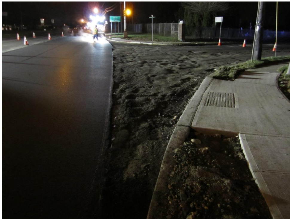
Figure 3 - Existing Pavement Condition at an Intersection of Route 184
