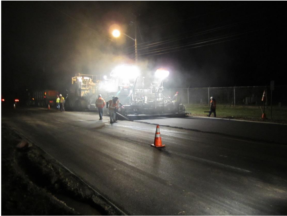
Figure 2 – HMA Paving on NJ Route 184
