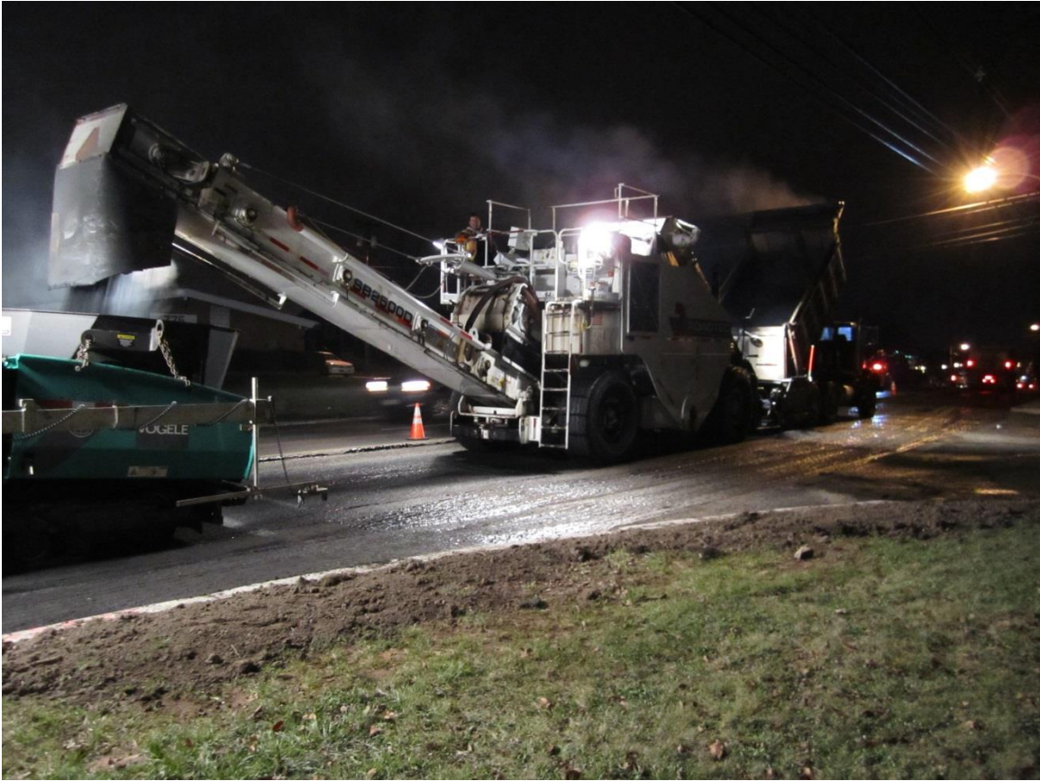
Figure 4 - Paving Train During Production (from Right to Left – Paver, Material Transfer Vehicle, and Delivery Truck)
