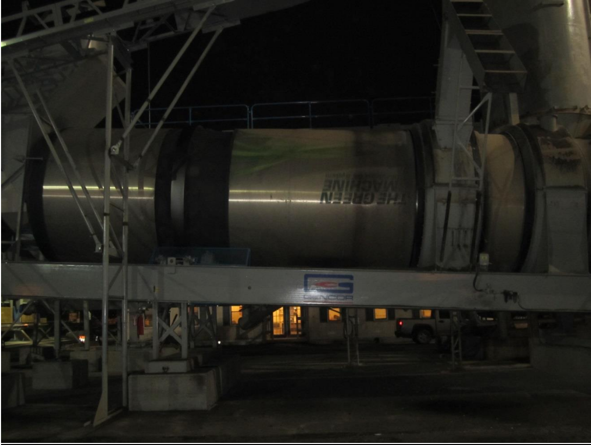
Figure 1 – Gencor Green Machine Modified Drum Plant
