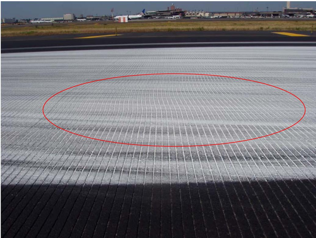
Figure 4.1 – Slipping at Newark Airport – Middle of Paving Lane
