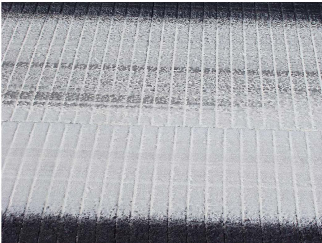
Figure 4.2 – Slipping at New Airport – Longitudinal Joint
