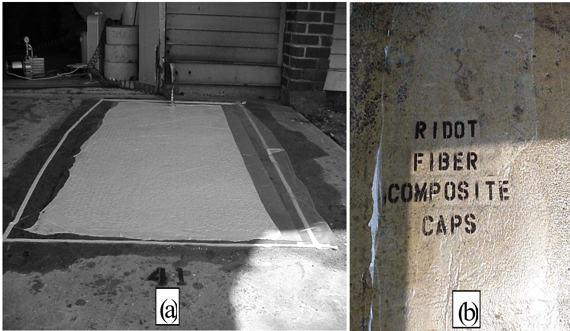
Figure 4.9: Full Scale Trial (A) During Vacuuming and (B) Finished Composite Surface
