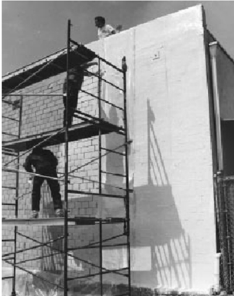
(a) Unreinforced masonry wall
