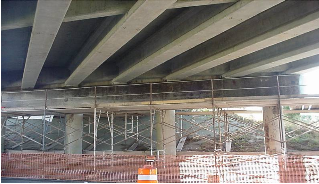
Figure 5.4: Scaffolding and safety measures
