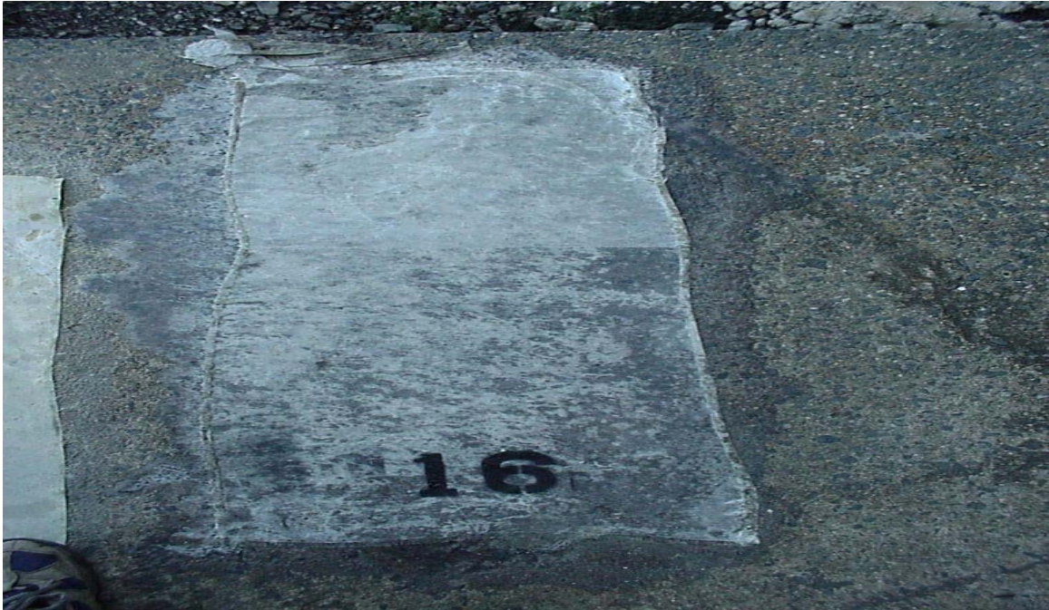
Figure 4.3: Sikadur® 35 Composite under Wet Conditions Two Days after Curing
