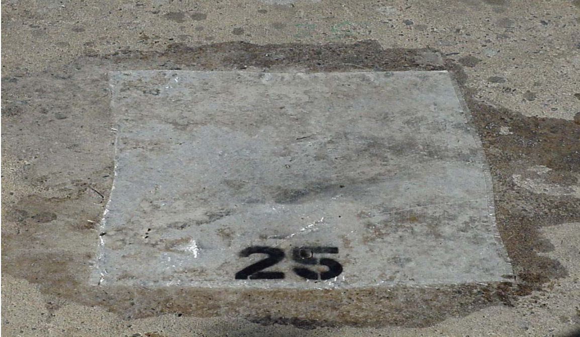
Figure 4.7: Sikadur ® Hex 300 Composite under Wet Conditions Two Days after Laminating
