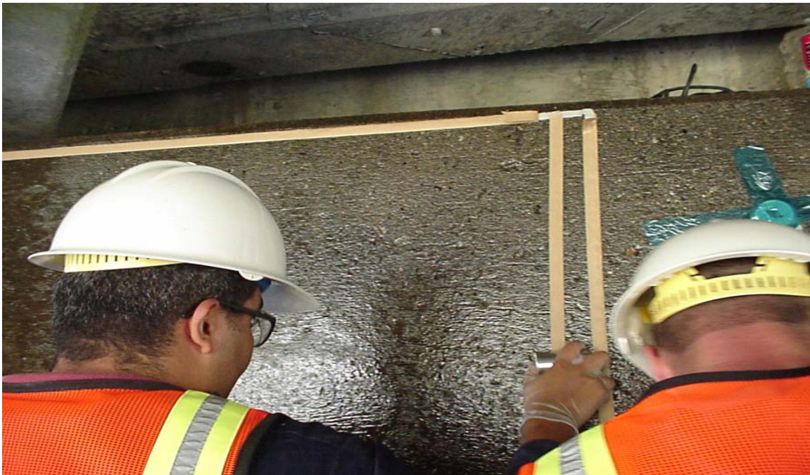
Figure5.7 : Application of Sealant Tape onto Primed Concrete Surface
