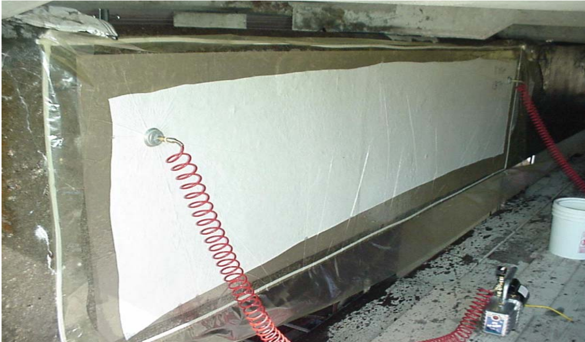
Figure 5.9 : Completed Vacuum Bagging System
