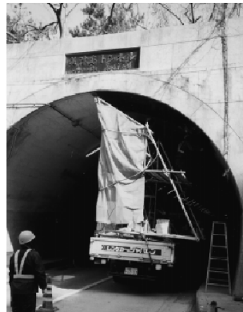
(b) Tunnel lining
