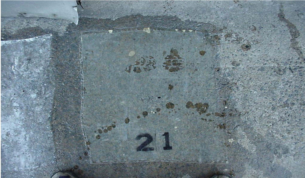
Figure 4.5: Sikadur® 35 Composite under Wet Conditions On the Day Three
