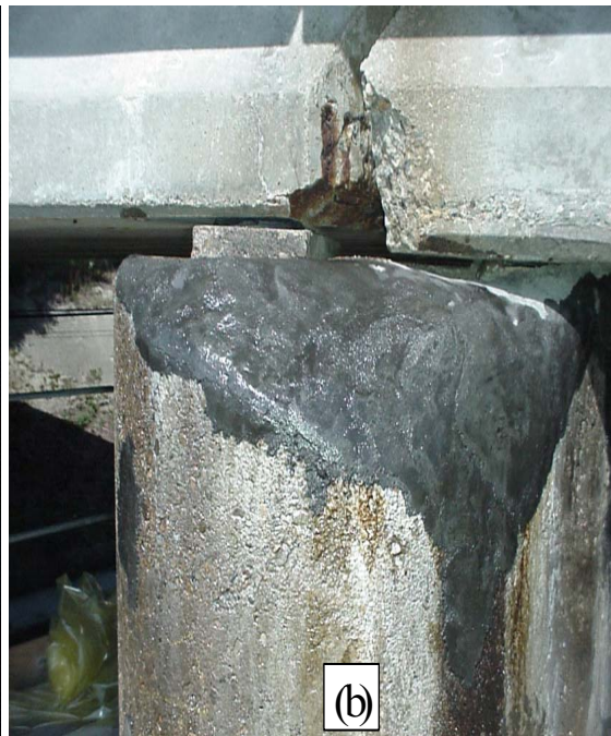
Figure 5.6 : (A) Wet Burlap Placed Over Freshly Placed Repair Mortar on Pier Cap End (B) Cured Repair Concrete on Pier Cap End
