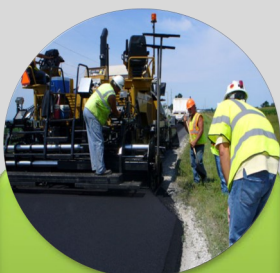
Roadway and Worker Safety
