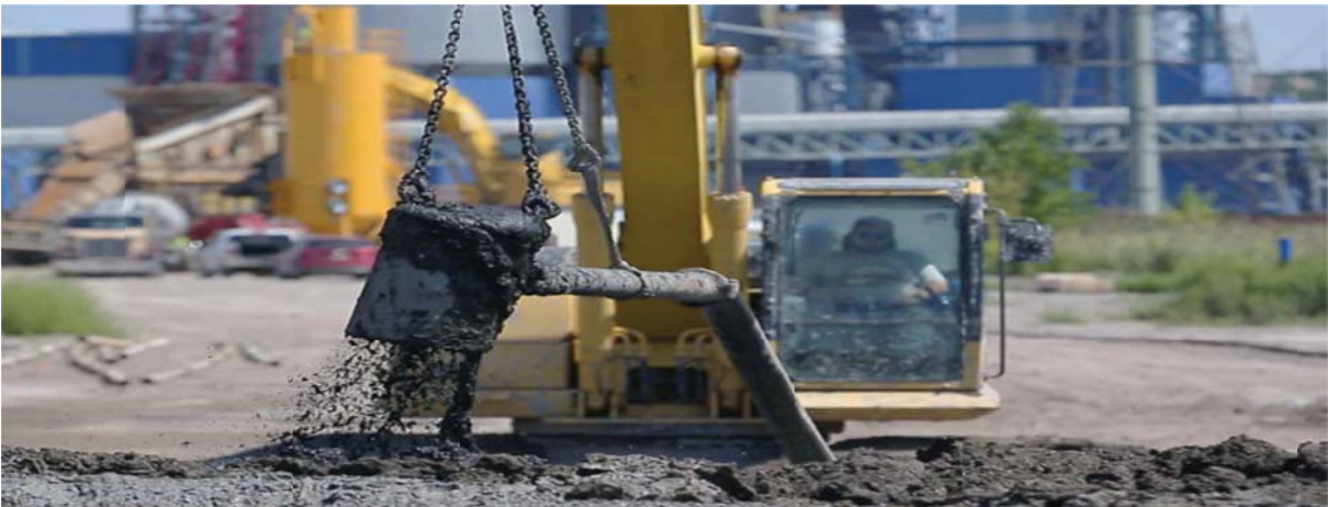
CAIT brought pneumatic tube mixing (PTM) to the United States for the first time and did a pilot project to quantify and validate it as an effective technique for our region. Photo: ©Drew Noel Photography/Rutgers CAIT.
