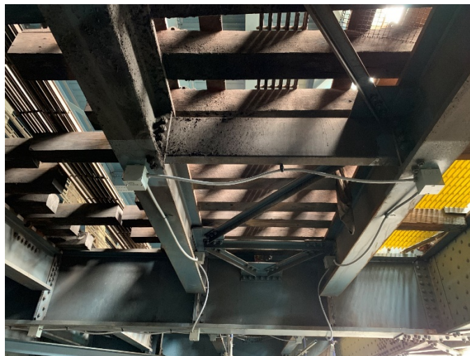
Figure 21 Sample layout of the SHM system
