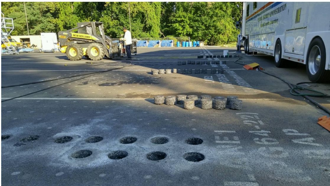
Figure 2 – Field Cores Recovered from FHWA ALF for Asphalt Mixture and Binder Testing
