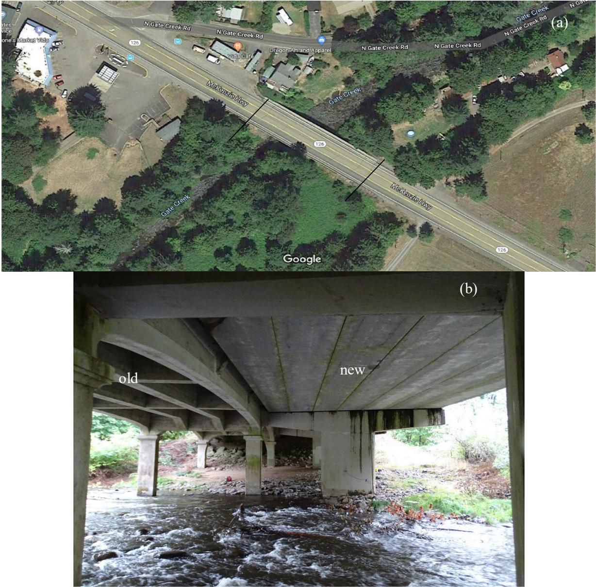
Fig. 1. (a) Tested bridge location and (b) old and new parts of the structure with different superstructures.
